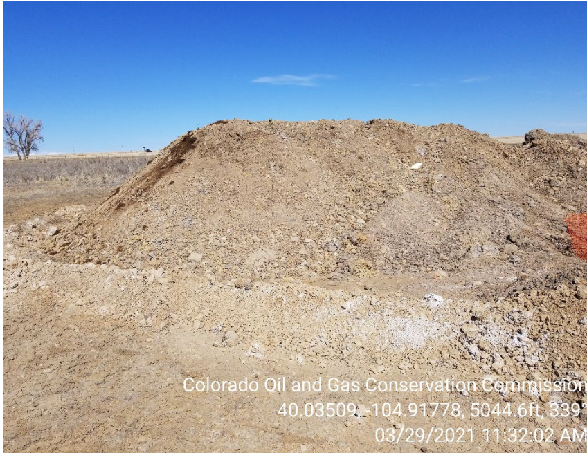
Photo 3 – Soils stored on site with inadequate BMPs
