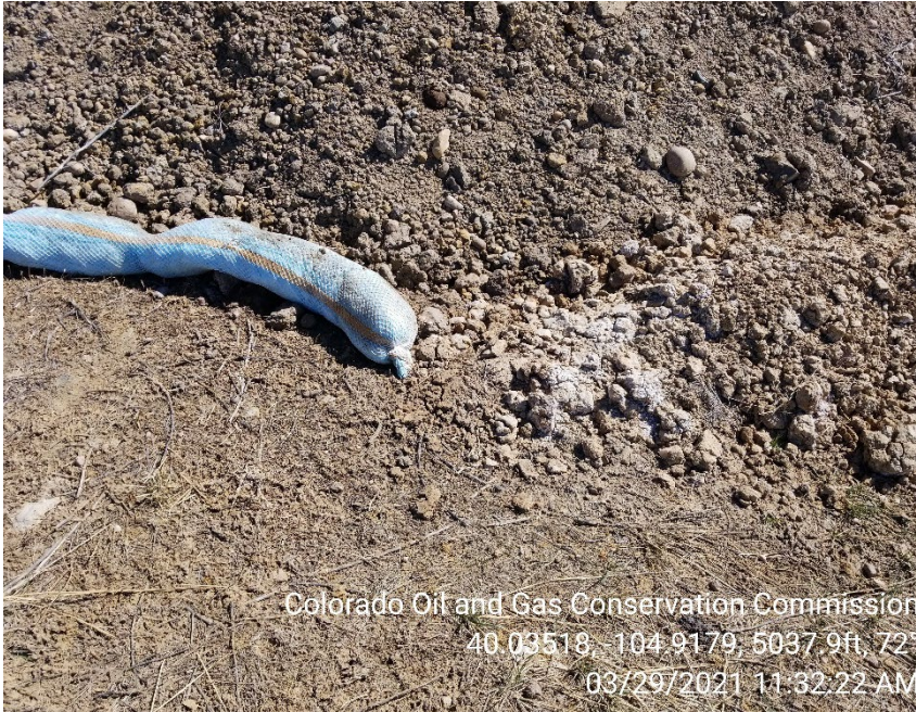
Photo 5 –Inadequate BMPs
