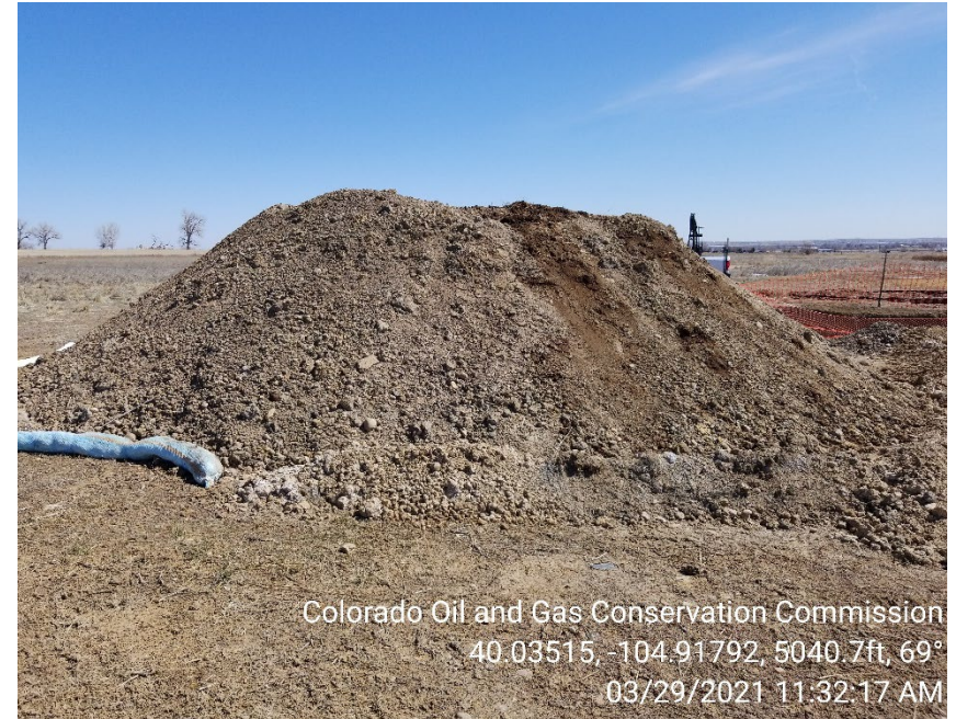
Photo 4 – Soils stored on site with inadequate BMPs
