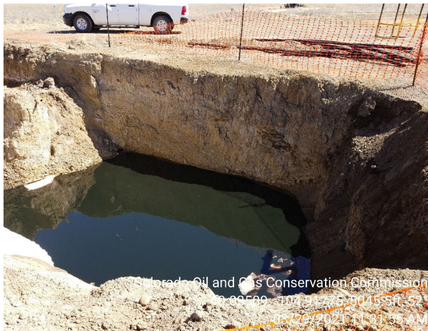
Photo 1 – Free product observed on groundwater in open excavation.
