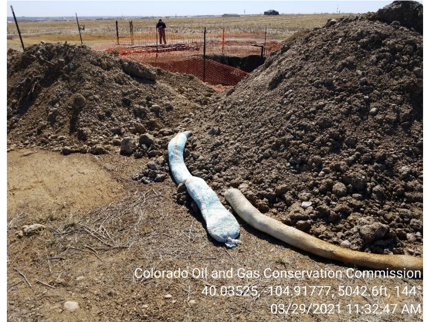
Photo 6 – Soils stored on site with inadequate BMPs
