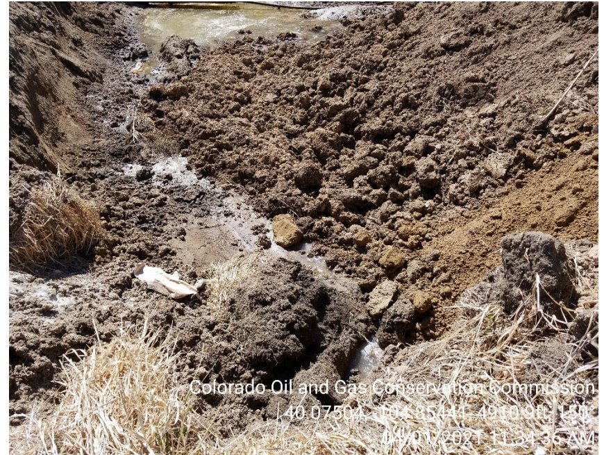
Photo 6 – Soil stockpile pushed back into open excavation.
