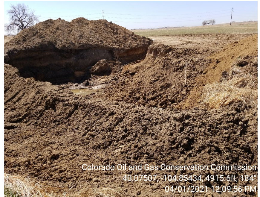
Photo 2 – Ditch wall. Fencing around open excavation has been removed.
