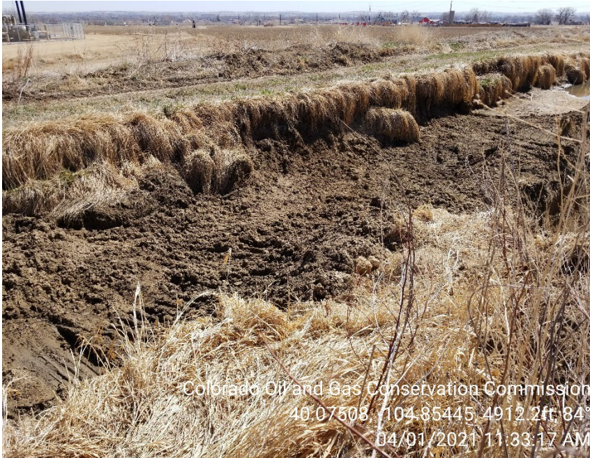
Photo 3 – Irrigation ditch floor has been scraped by excavator since last inspection.
