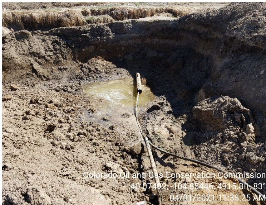
Photo 9 – Groundwater with hydrocarbon sheen observed in open excavation.
