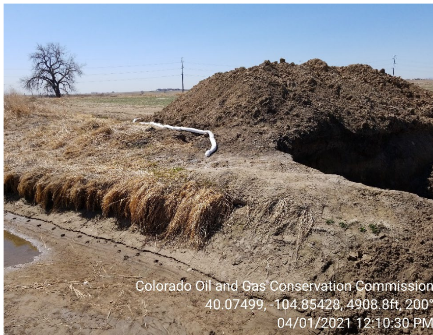
Photo 13 –BMPs inadequate to contain runoff; any runoff from the eastern portion of the soils stockpile would go into irrigation ditch.
