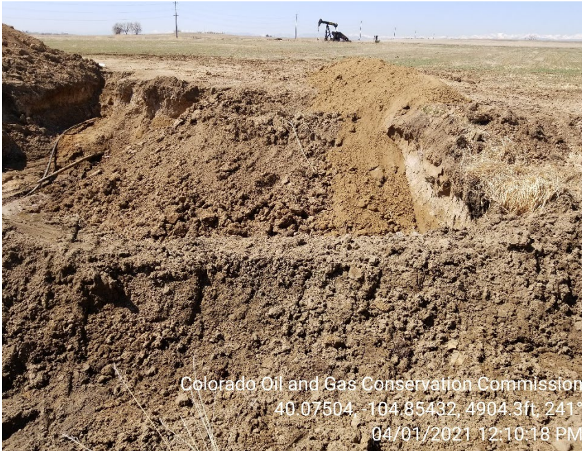
Photo 5 – Clean fill on location. One soil stockpile appears to have been pushed back into open excavation.
