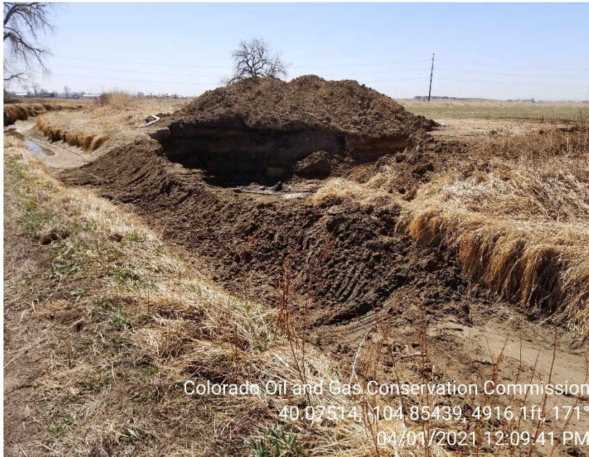
Photo 1 – Wall of Brantner Irrigation ditch during 4/1/2021 inspection; work to reconstruct wall had begun since previous inspection. Work appear to still be in progress.
