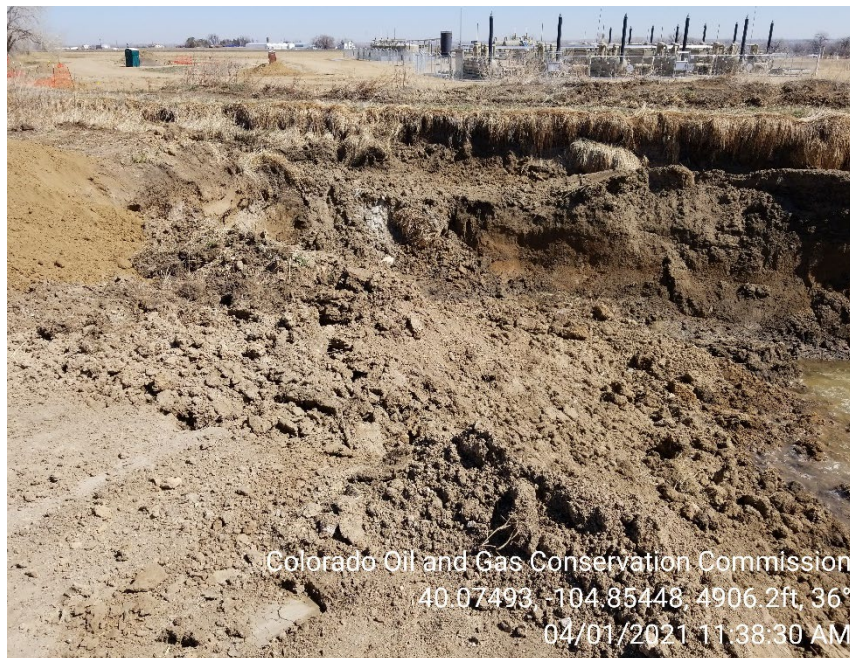
Photo 7 – Soil stockpile pushed back into open excavation.
