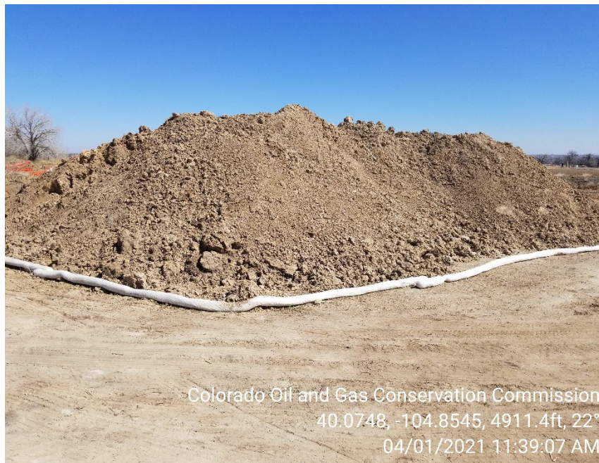
Photo 11 – Soils stored on location; BMPs inadequate to contain runoff
