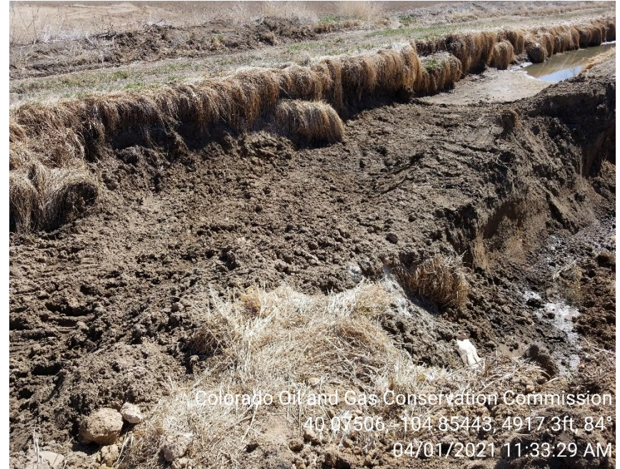
Photo 4 – Collapsed wall of Brantner Irrigation ditch with scraped portions of ditch floor.
