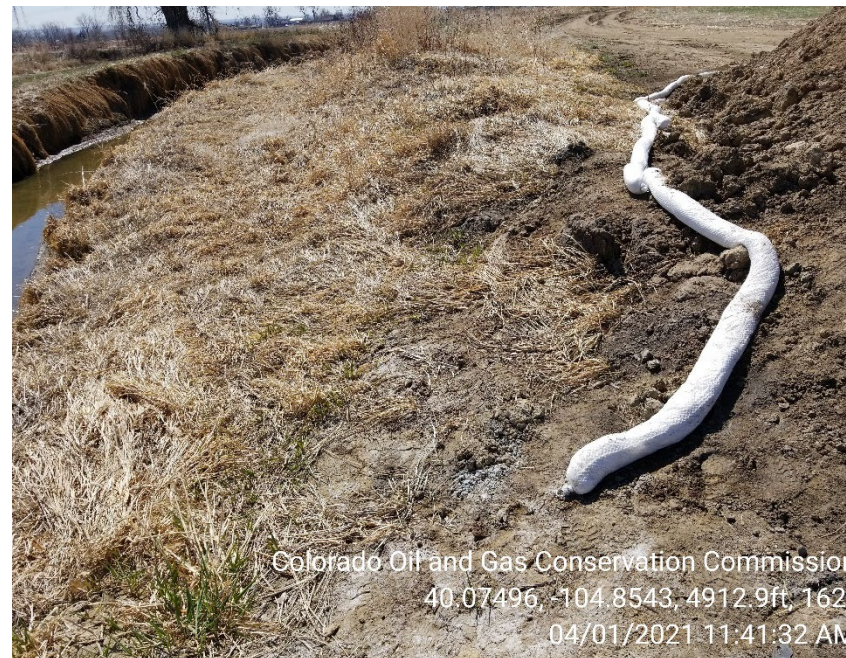
Photo 12 – Soils stored on location; BMPs inadequate to contain runoff
