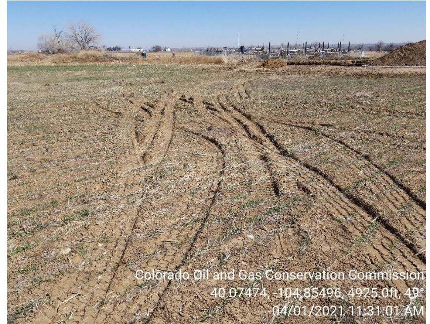
Photo 16 – Vehicle tracking has extended an additional ~150' west of the excavation, making ruts in field
