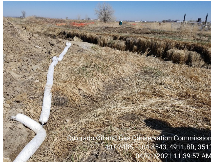
Photo 14 – BMPs inadequate to contain runoff
