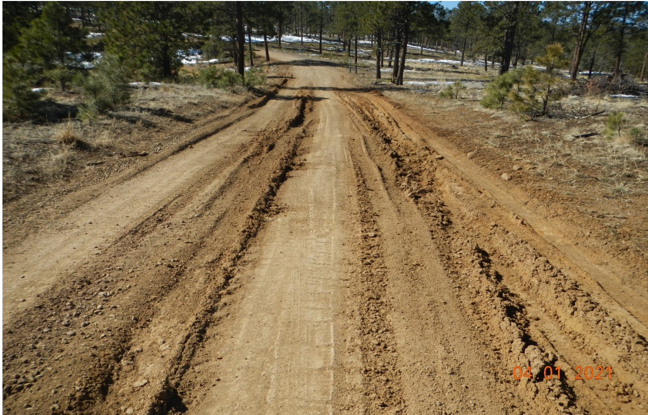
Photo 2. There is vehicle rutting along the main road traveling southwest toward the location.
