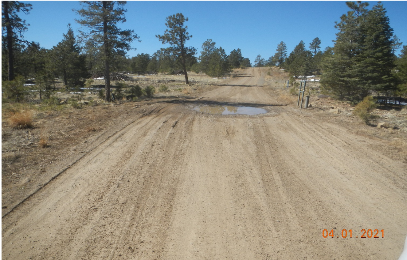
Photo 1. Facing southwest along the main road. Vehicles are driving around where water is accumulating in the road causing widening of the road. This area needs to be repaired.
