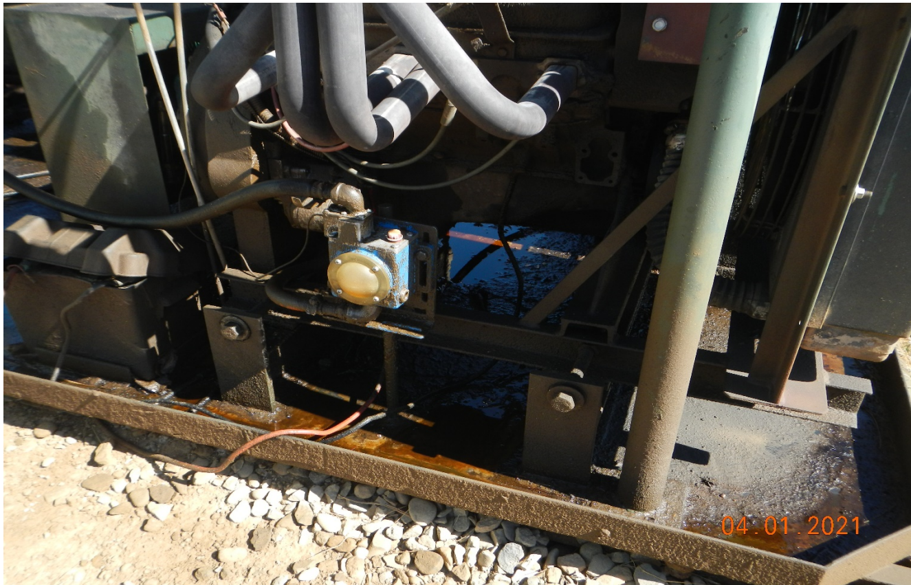
Photo 5. There is still oil inside the engine skid that needs to be cleaned up.
