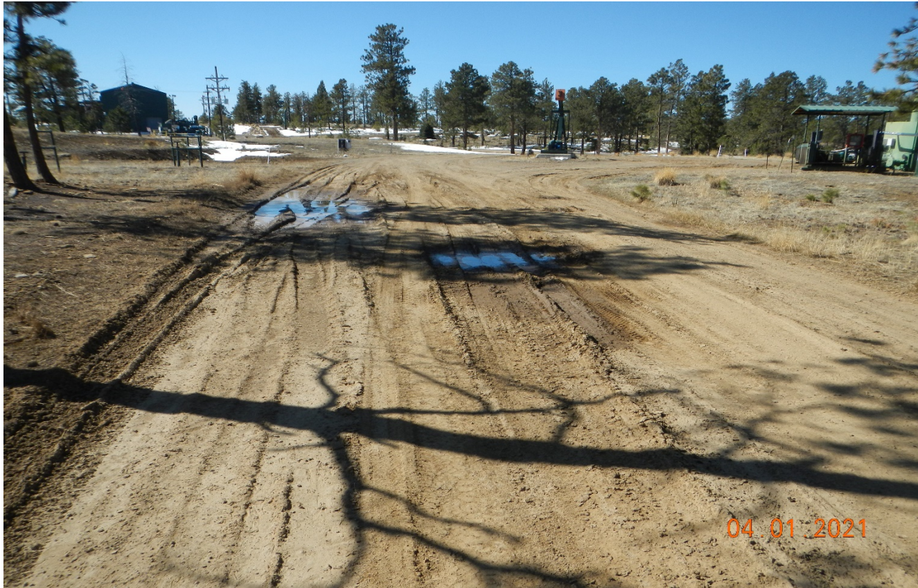
Photo 3. Facing southwest along the main road near the location. Vehicles have caused widening of the road and causing damage outside of road boundary. Vehicles shall not travel outside of access road boundary per rule 1002.e(4).
