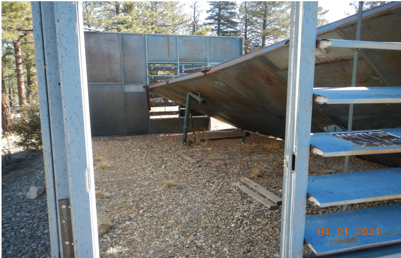
Photo 3. The wall panel is leaning on the pipe riser. Pipe riser are not LOTO.
