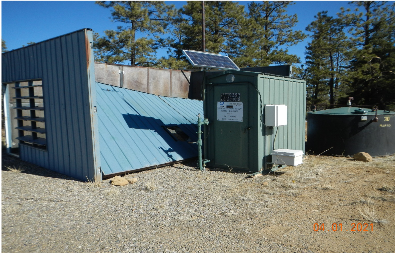
Photo 2. The wall panel near the meter shed has fallen over.
