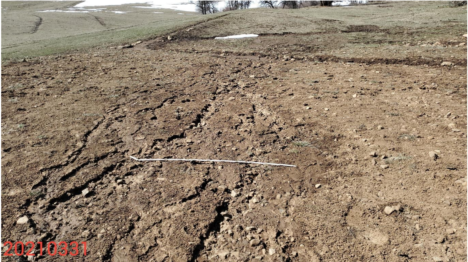
Photo 16: Photo taken from the western areas of the Location, facing west. Photo shows control measures to protect and stabilize the Location remain missing or insufficient; ditch has filled with sediment; erosion degradation evident; off-site sediment transport evident. 6 foot measuring stick used for reference.
