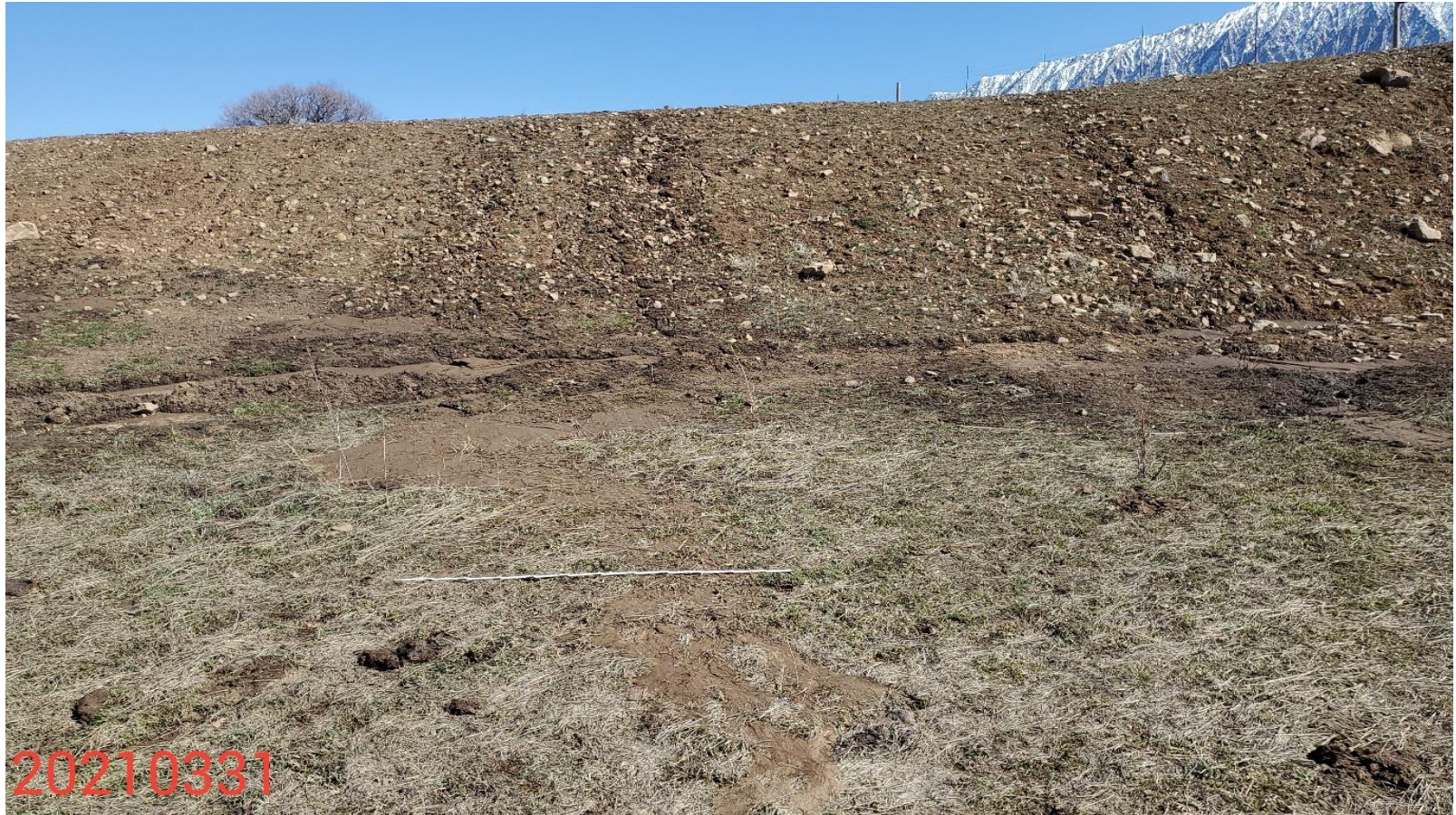
Photo 20: Photo taken from the southwest of the Location, facing northeast. Photo shows control measures to protect and stabilize the Location remain missing or insufficient; erosion degradation evident; photo also shows sediment has filled an irrigation ditch, and has been transported off-site. 6 foot measuring stick for reference.
