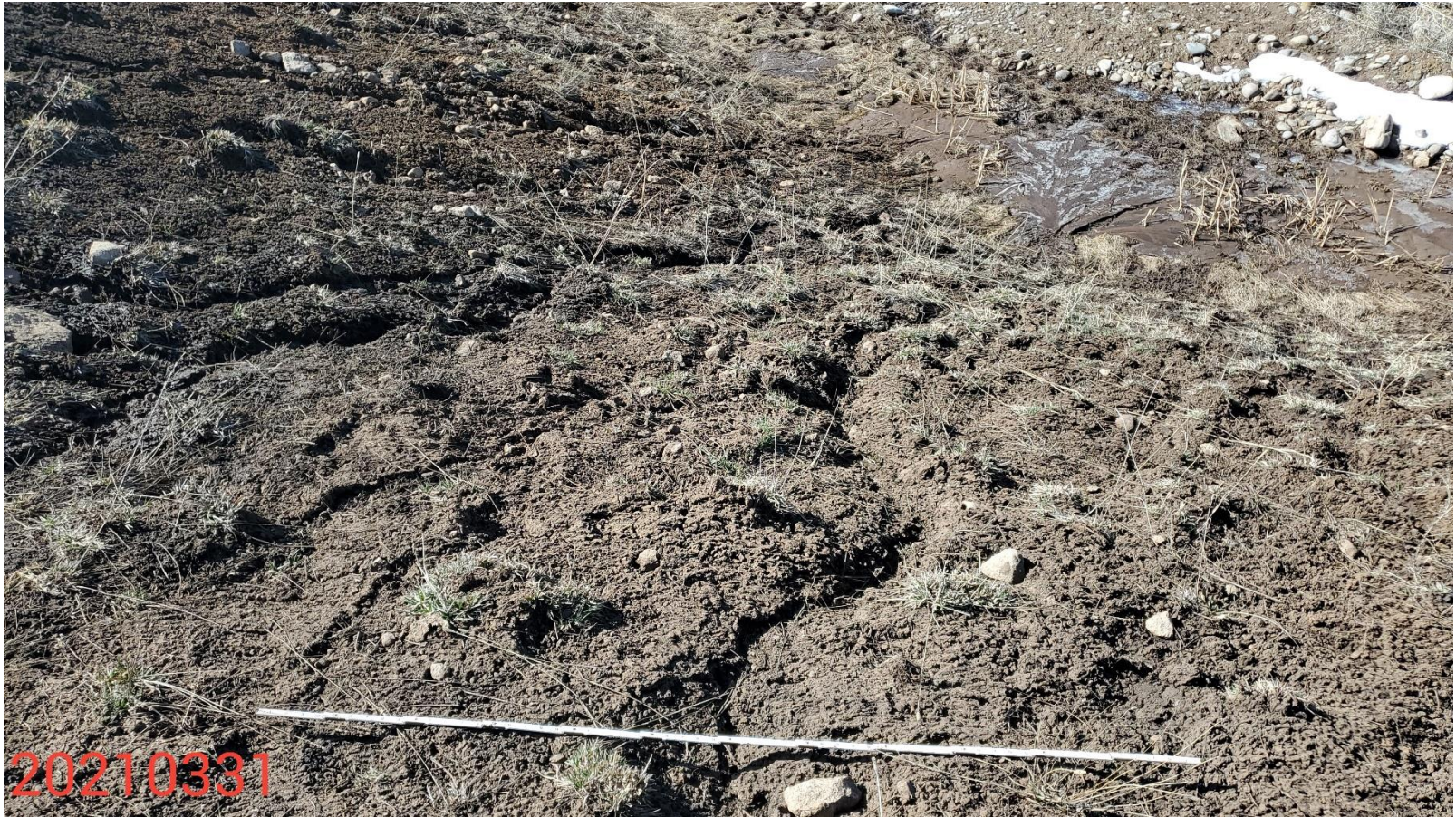
Photo 5: Photo taken from the northeast corner of the Location, facing southwest. Photo shows control measures to protect and stabilize the Location remain missing or insufficient; erosion degradation evident. 6 foot measuring stick for reference.
