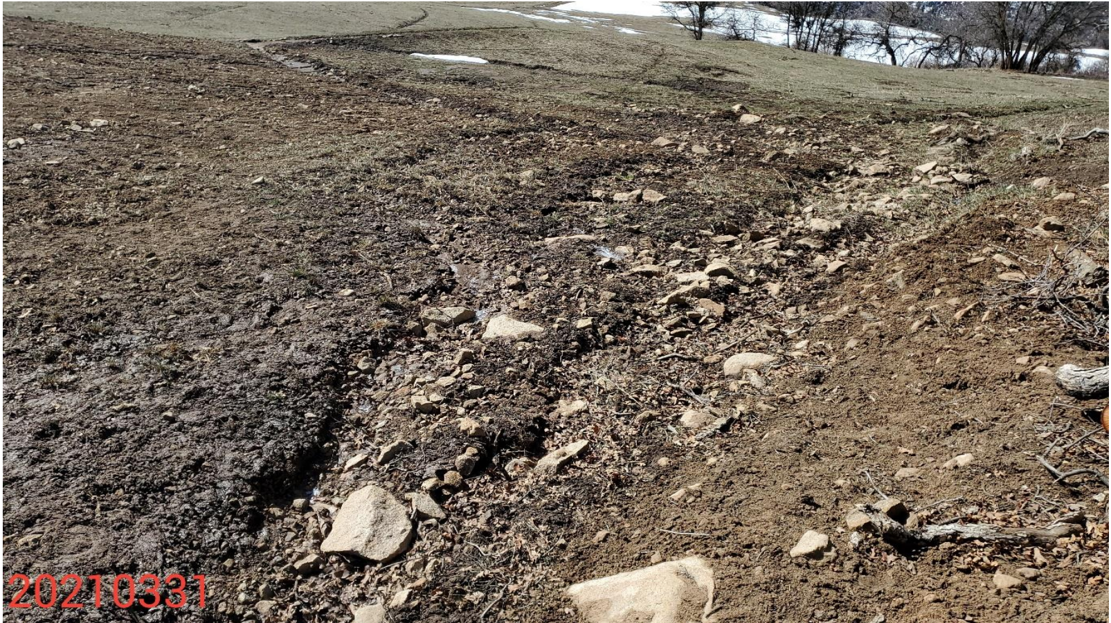
Photo 14: Photo taken from the northwestern end of the Location, facing southwest. Photo shows stormwater ditch BMPs have not been constructed in accordance with good engineering practices, including an appropriate outlet to allow for sediment laden-free stormwater discharge; erosion degradation evident.
