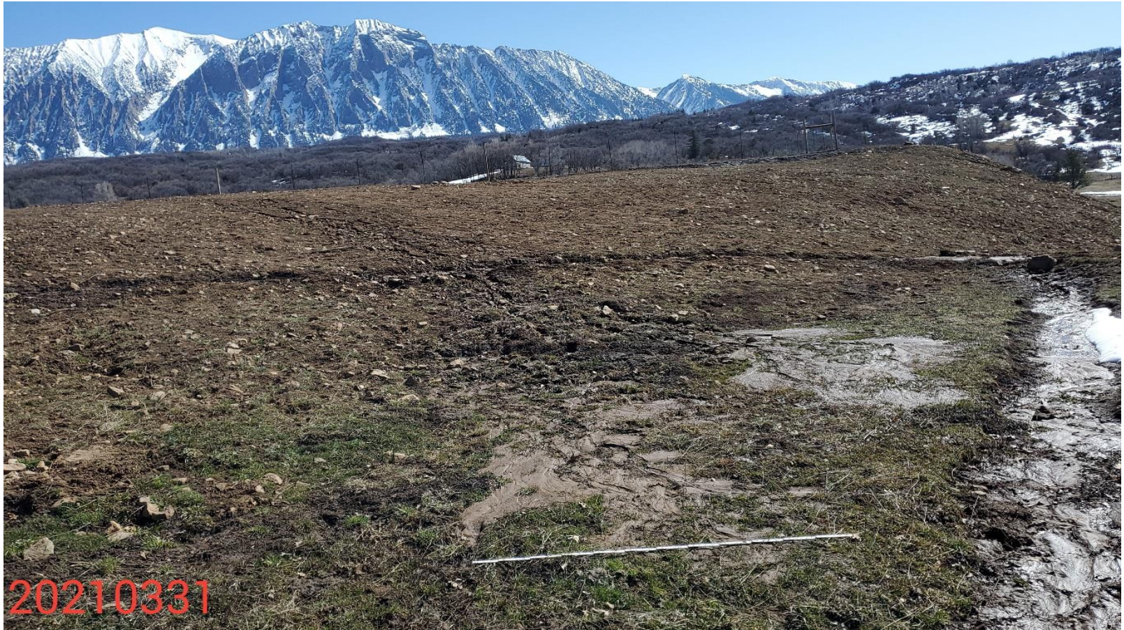
Photo 15: Photo taken from the western end of the Location, facing east. Photo shows control measures to protect and stabilize the Location remain missing or insufficient; ditch has filled with sediment; erosion degradation evident; off-site sediment transport evident. 6 foot measuring stick used for reference.
