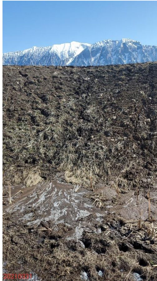
Photo 6: Photo taken from the northeast corner of the Location, at the toe of the cut slope, facing northwest. Photo shows control measures to protect and stabilize the Location remain missing or insufficient; erosion degradation evident.
