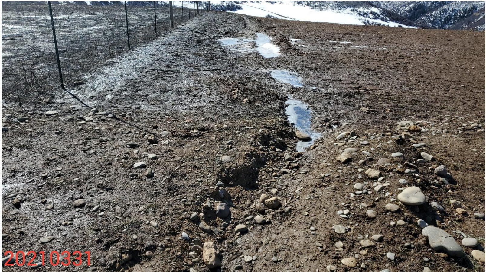
Photo 13: Photo taken from the west end of the Location. Photo shows the stormwater ditch has not been constructed in accordance with good engineering practices; ditch filled with sediment.
