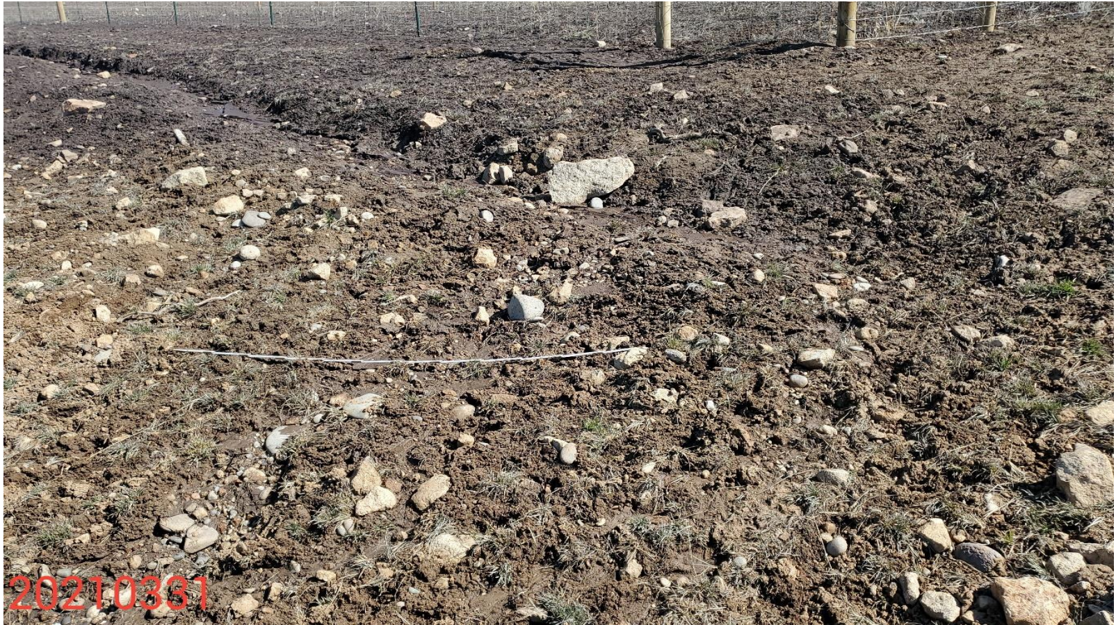
Photo 17: Photo taken from the stormwater ditch on the southwest corner of the pad. Photo shows stormwater ditch BMP has not been constructed in accordance with good engineering practices, including an appropriate outlet to allow for sediment laden-free stormwater discharge.
