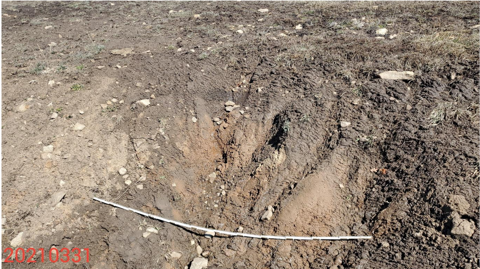
Photo 9: Continued from photo 8. Photo shows control measures to protect and stabilize the Location remain missing or insufficient; erosion degradation evident. 6 foot measuring stick for reference.
