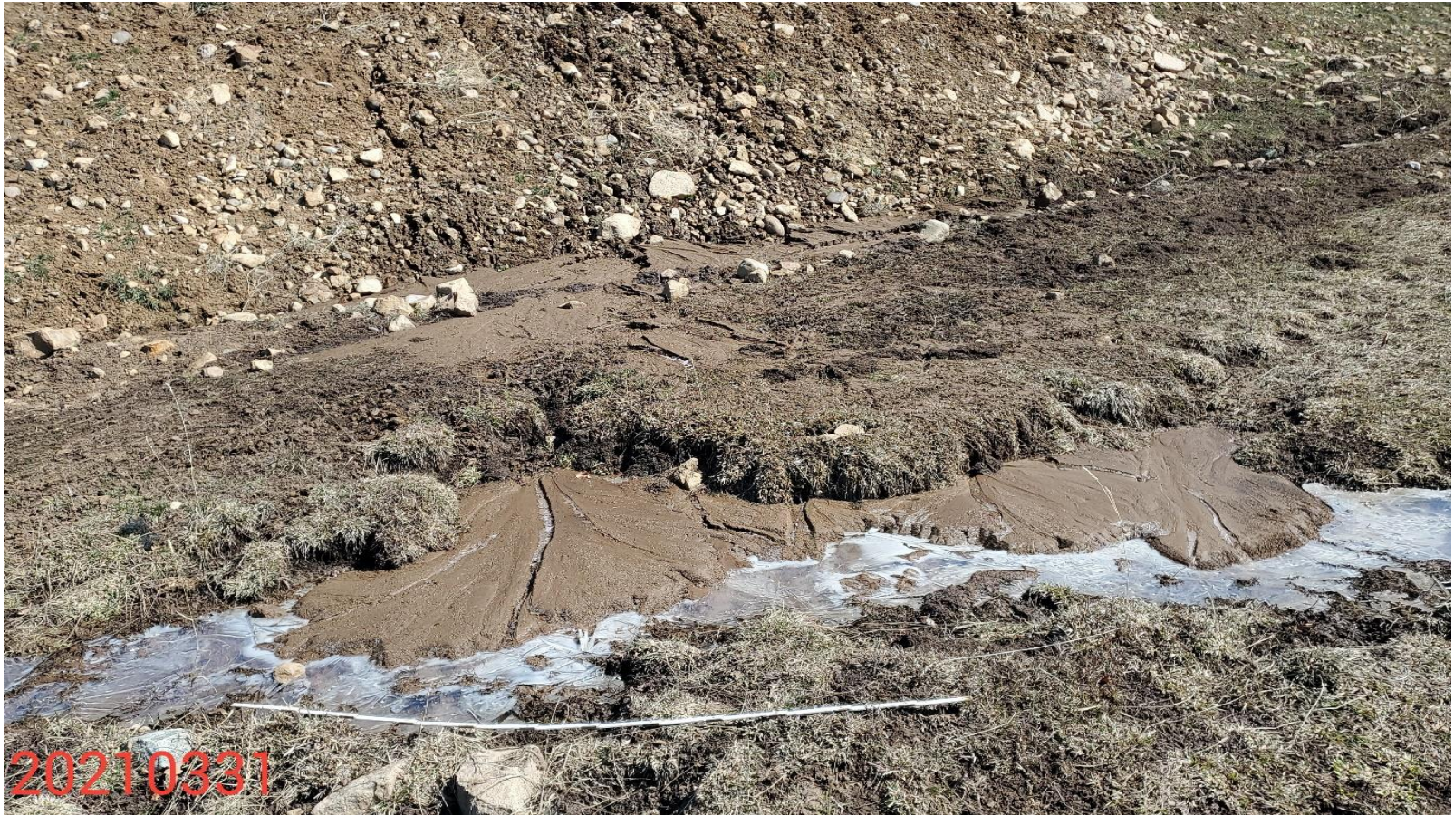
Photo 21: Photo shows off-site sediment discharge on the southwest end of the Location. 6 foot measuring stick for reference.
