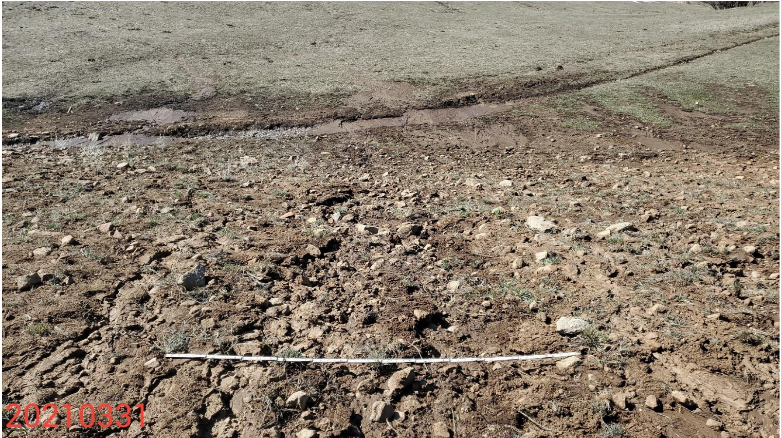
Photo 18: Photo taken from the slopes below the end of the ditch observed in photo 17. Photo shows an appropriate outlet to allow for sediment laden-free stormwater discharge has not been constructed at the ditch in accordance with good engineering practices. Photo also shows control measures to protect and stabilize the Location remain missing or insufficient; erosion degradation and off-site sediment transport evident.
