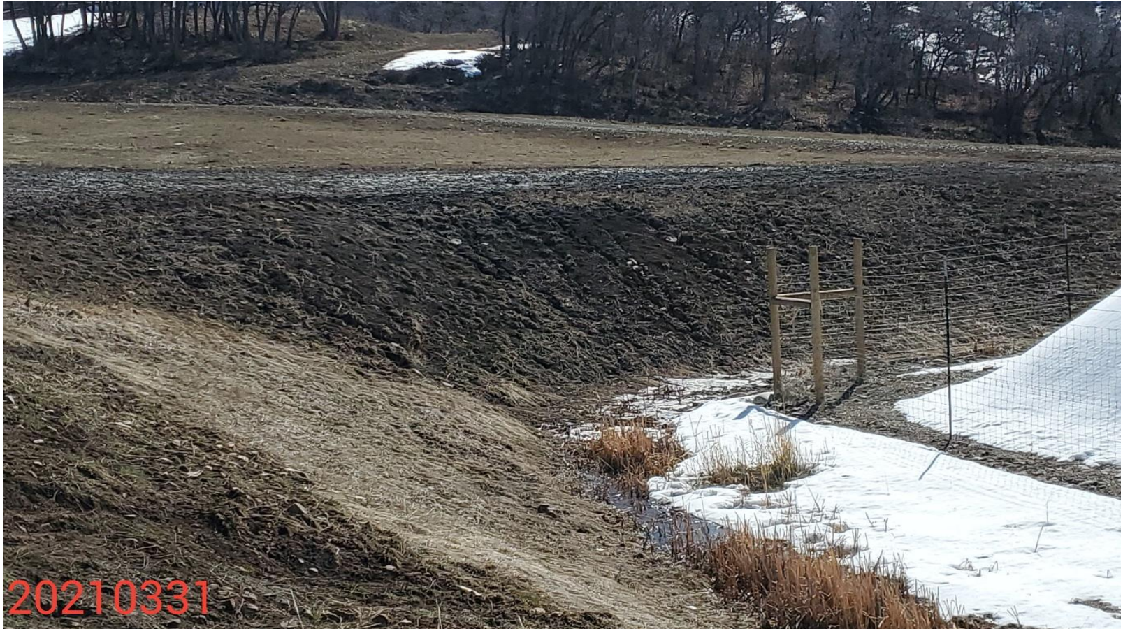
Photo 7: Photo taken from the northeast end of the Location, facing southeast. Photo shows cut slopes observed in photos 4-6. Photo shows control measures to protect and stabilize the Location remain missing or insufficient; erosion degradation evident.
