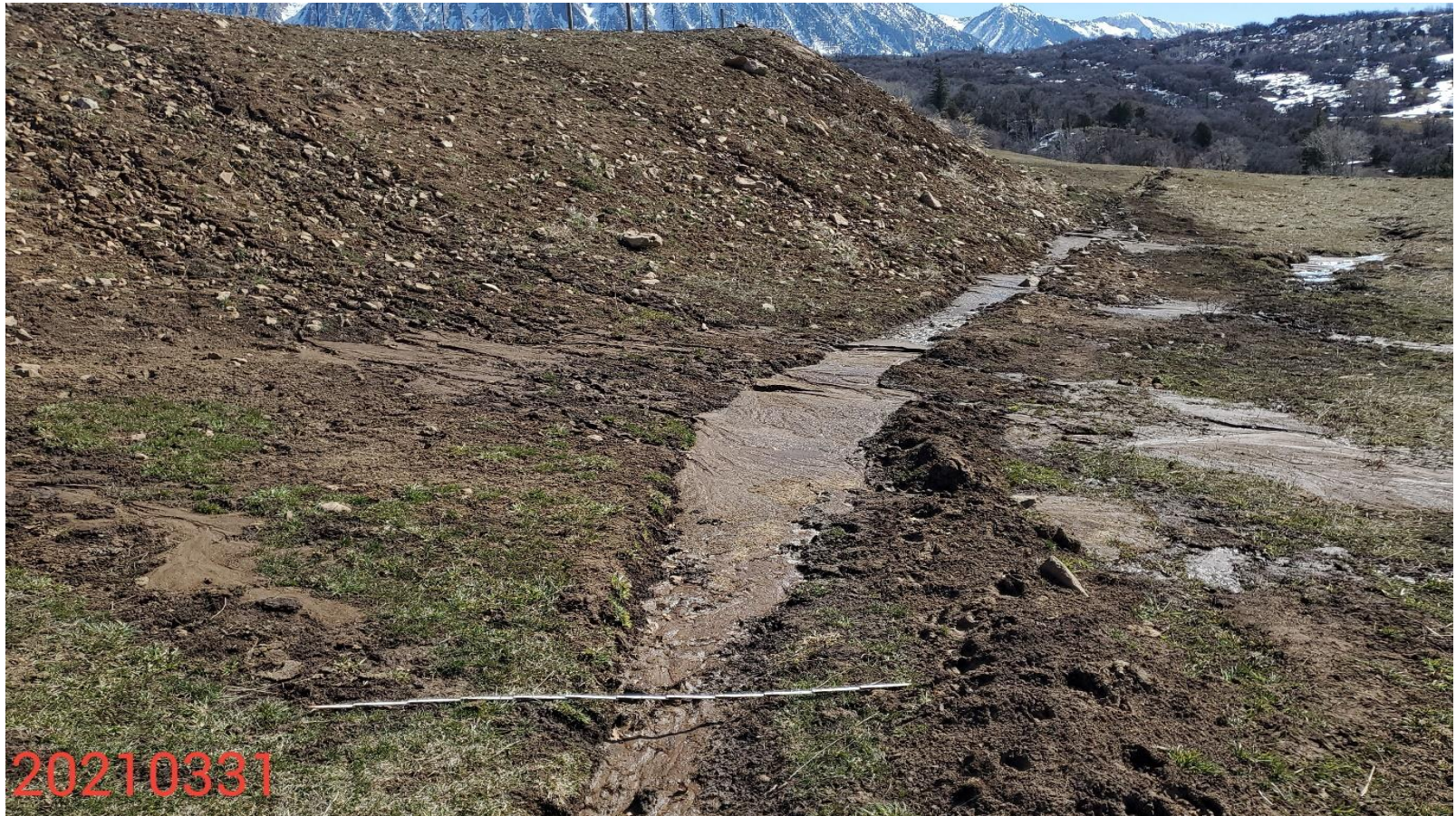
Photo 19: Photo taken from the irrigation ditch on the southwestern end of the Location. Photo shows control measures to protect and stabilize the Location remain missing or insufficient; photo also shows sediment has been discharged from the location, has filled the irrigation ditch and transported off-site. 6 foot measuring stick for reference.
