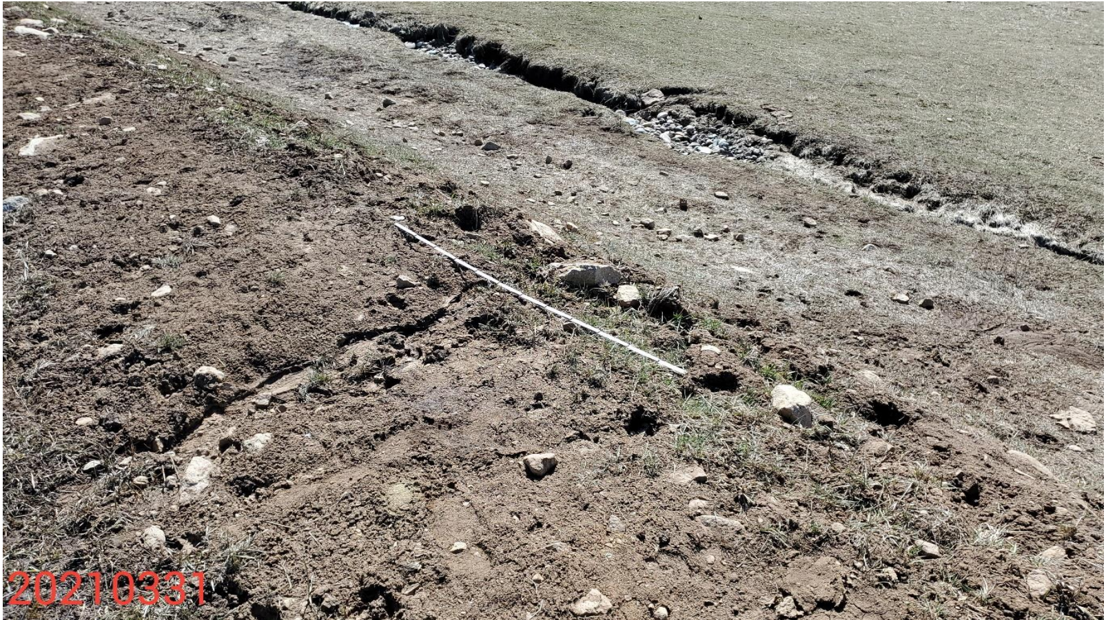
Photo 23: Photo taken from the south end of the Location, facing southeast. Photo shows erosion degradation due to runoff from the Location is now evident on the southern fill slopes. 6 foot measuring stick for reference.
