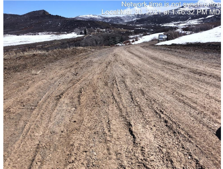
Photo #3343 No form of tracking control at entrance to location.
