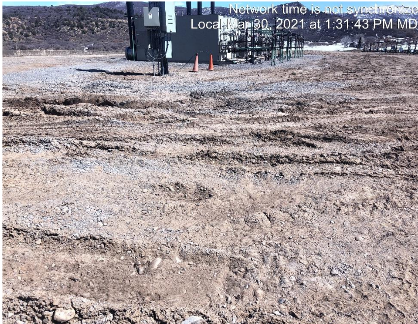
Photo #3339 Location lacks stabilization
