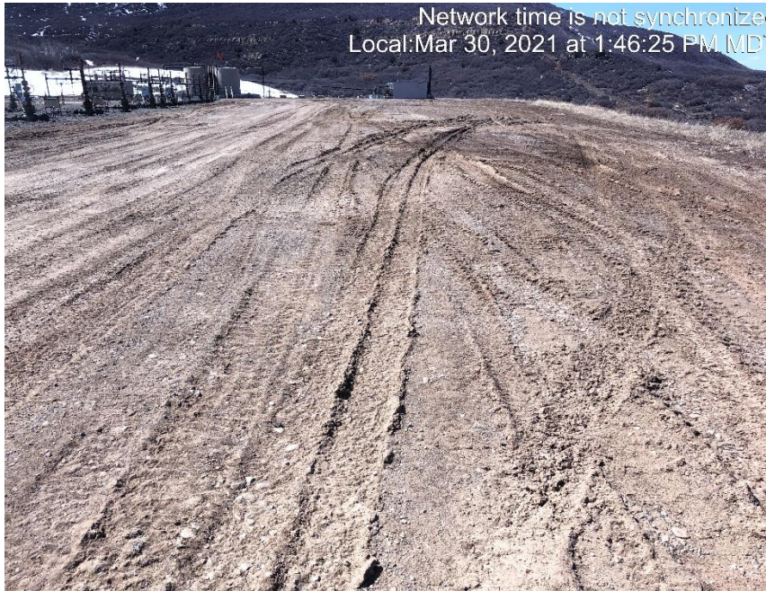
Photo #3342 Location lacks stabilization
