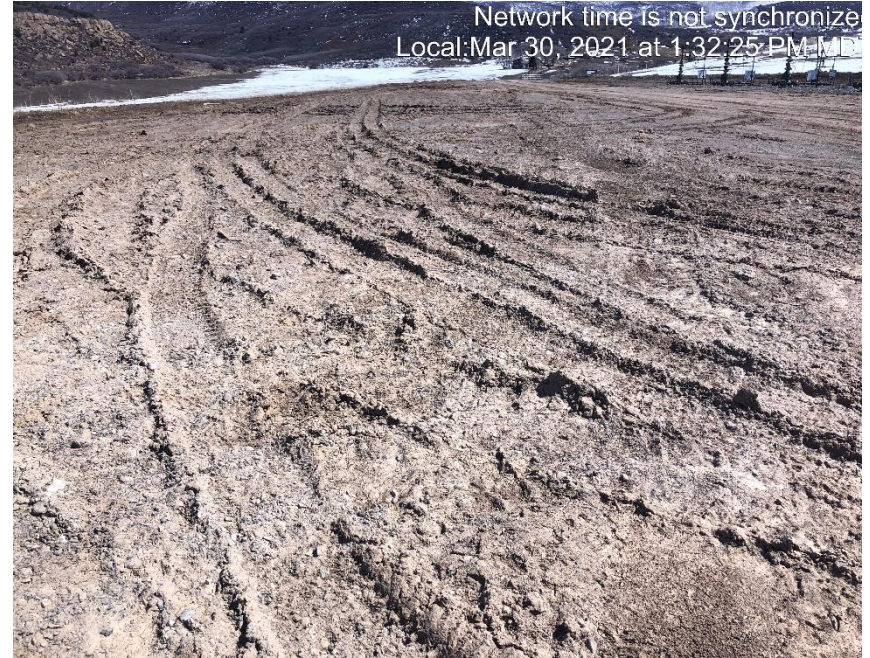
Photo #3340 Location lacks stabilization
