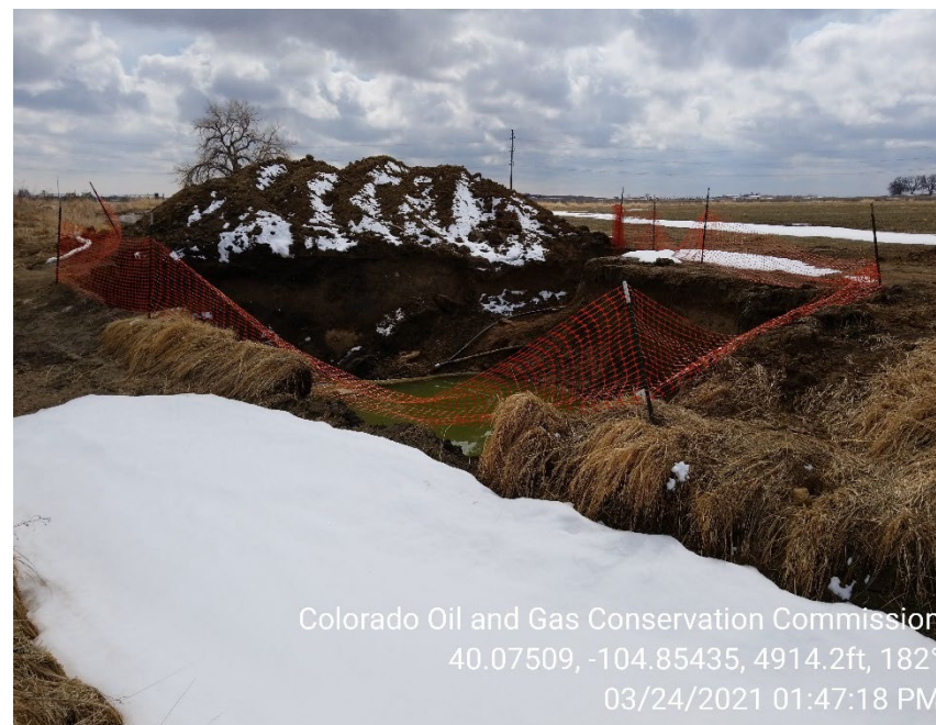
Photo 2 – Collapsed wall of Brantner Irrigation ditch during 3/24/2021 inspection.
