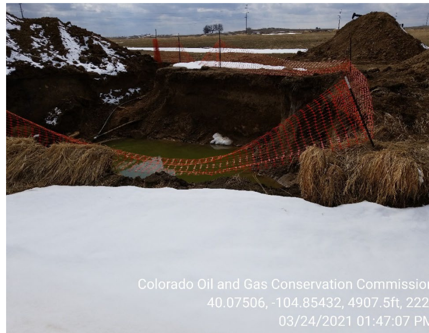
Photo 4 – Collapsed wall of Brantner Irrigation ditch during 3/24/2021 inspection.
