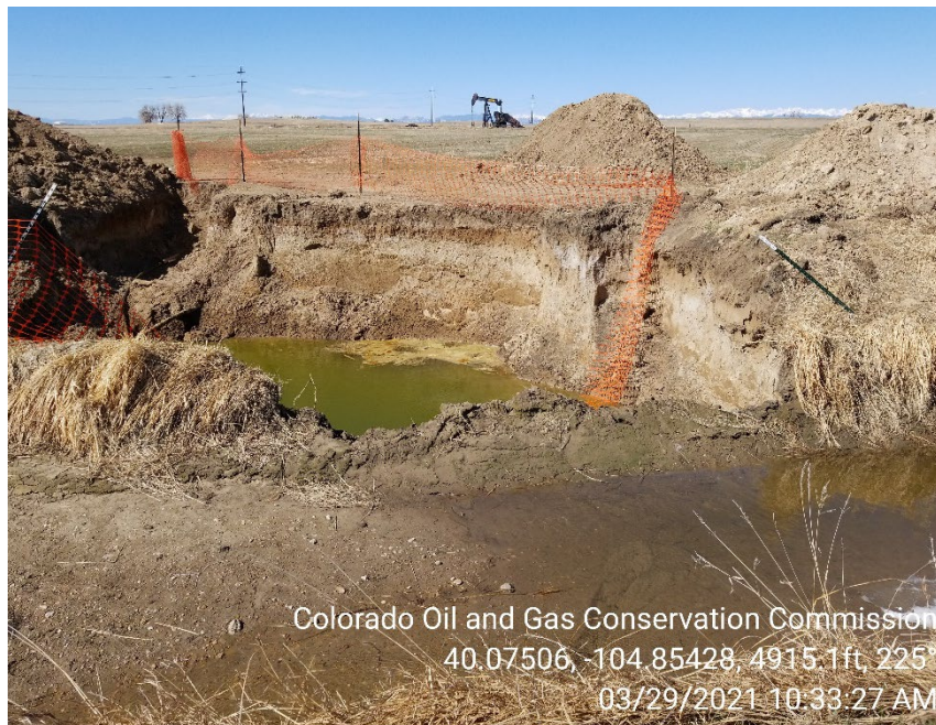
Photo 3 – Collapsed wall of Brantner Irrigation ditch during 3/29/2021 inspection. Fencing down around portions of the open excavation.
