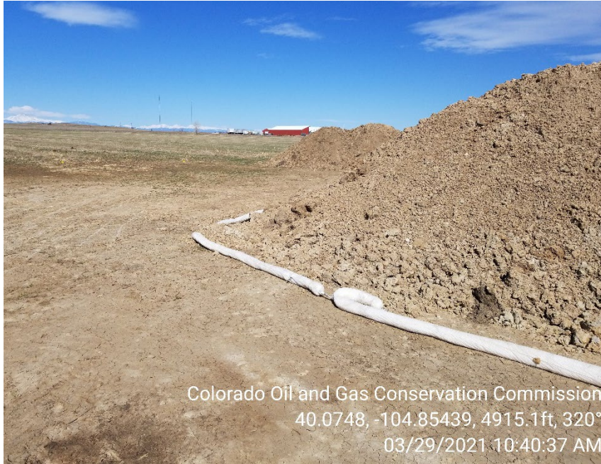
Photo 11 –BMPs inadequate to contain runoff
