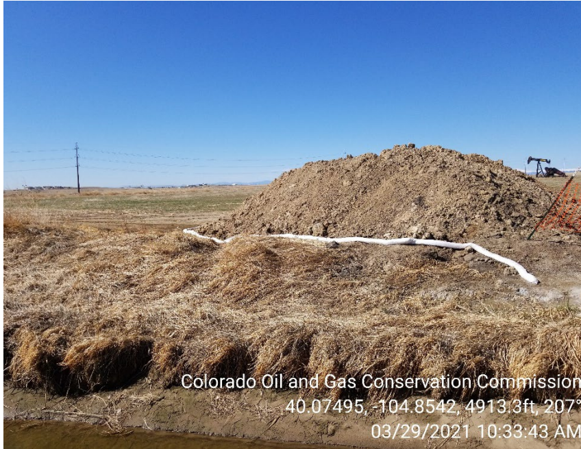
Photo 9 – Soils stored on location; BMPs inadequate to contain runoff
