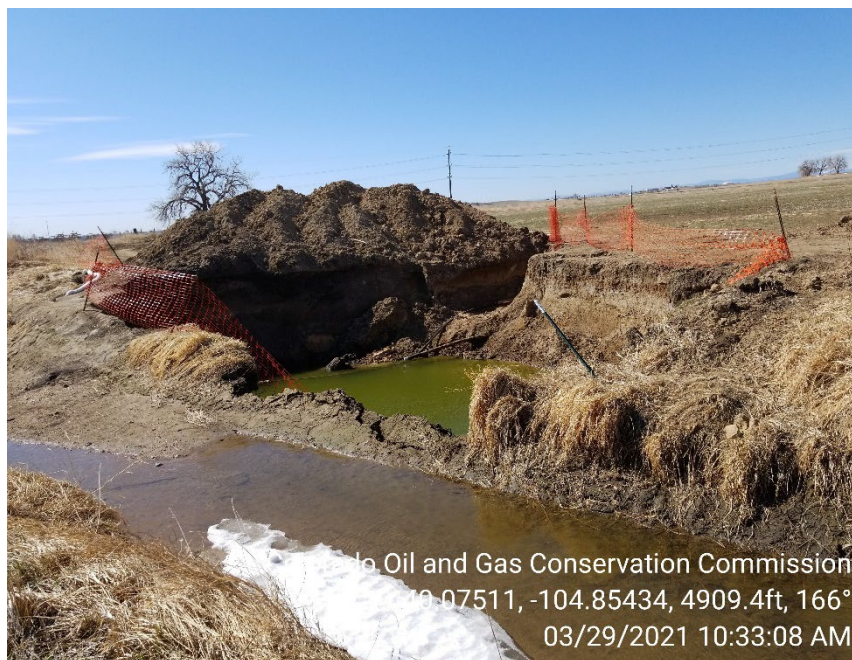
Photo 1 – Collapsed wall of Brantner Irrigation ditch during 3/29/2021 inspection. Additional collapse of the ditch wall has occurred since 3/24/2021 inspection.
