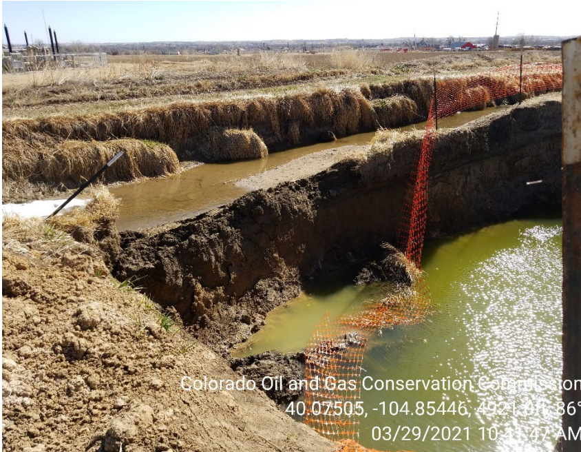
Photo 7 – Collapsed wall of Brantner Irrigation ditch during 3/29/2021 inspection. Fencing has fallen into open excavation. Groundwater observed in excavation.
