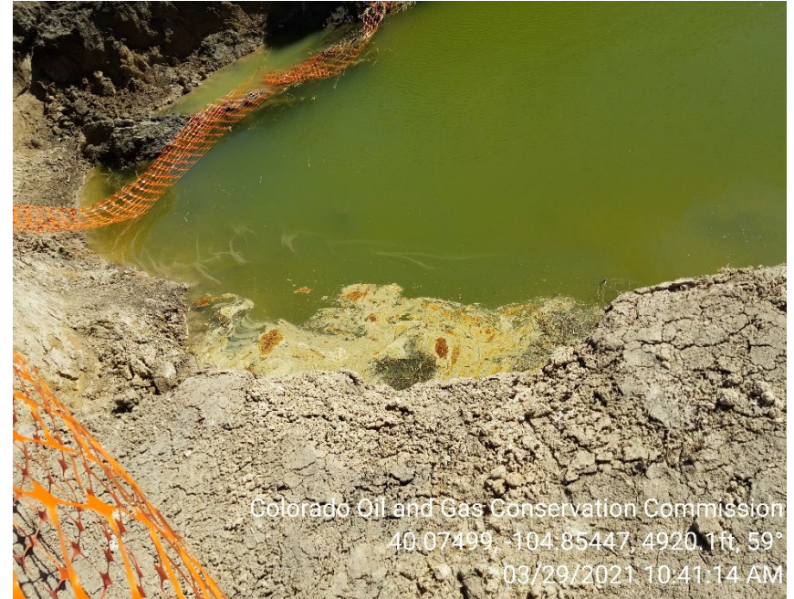
Photo 8 – Groundwater and sludge observed in open excavation.
