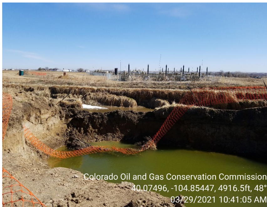
Photo 5 – Collapsed wall of Brantner Irrigation ditch during 3/29/2021 inspection.
