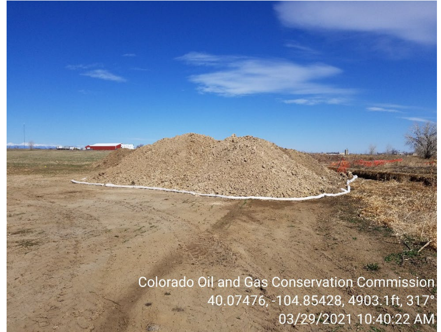
Photo 10 – Soils stored on location; BMPs inadequate to contain runoff
