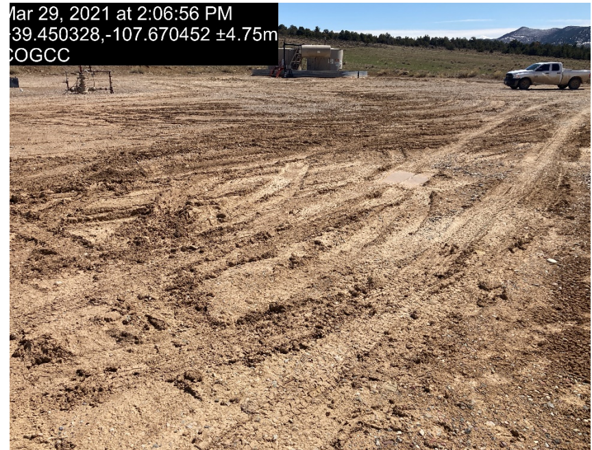
Lack of stabilization/compaction
