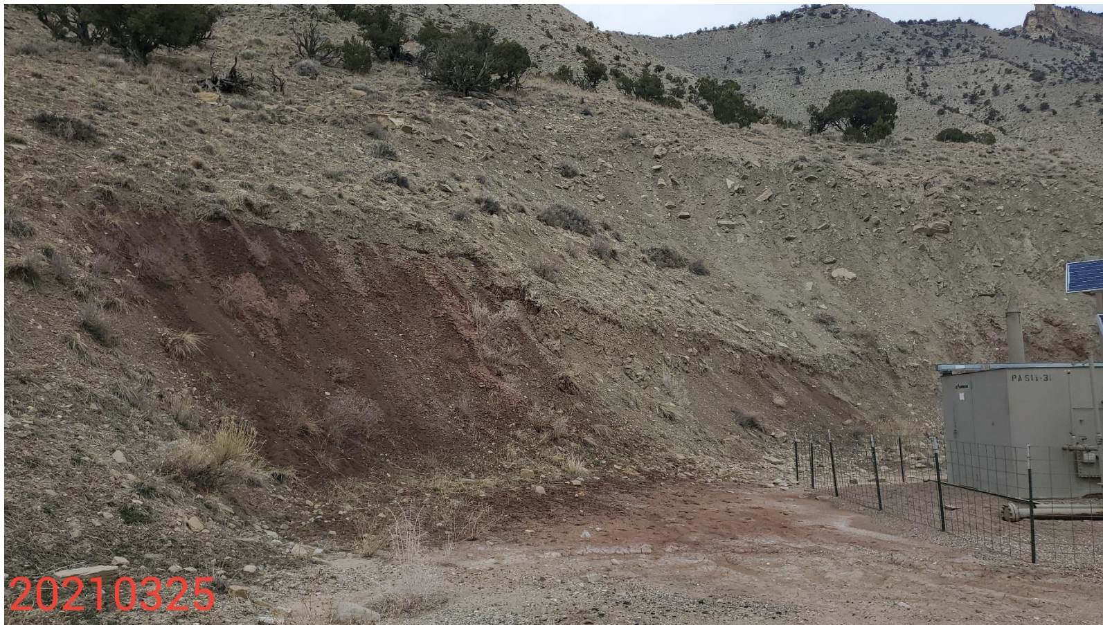
Photo 1: Photo taken from the northwest end of the Location, facing north. Photo shows that control measures to stabilize/protect the cut/fill slopes of the Location are missing or insufficient
