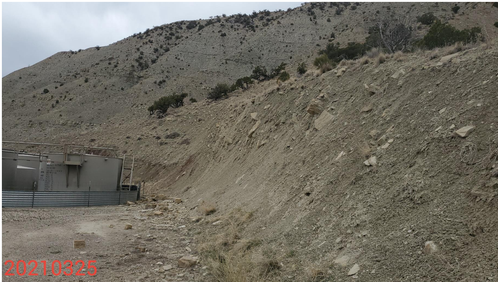
Photo 5: Photo taken from the northeast end of the Location, facing west. Photo shows that control measures to stabilize/protect the cut/fill slopes of the Location are missing or insufficient
