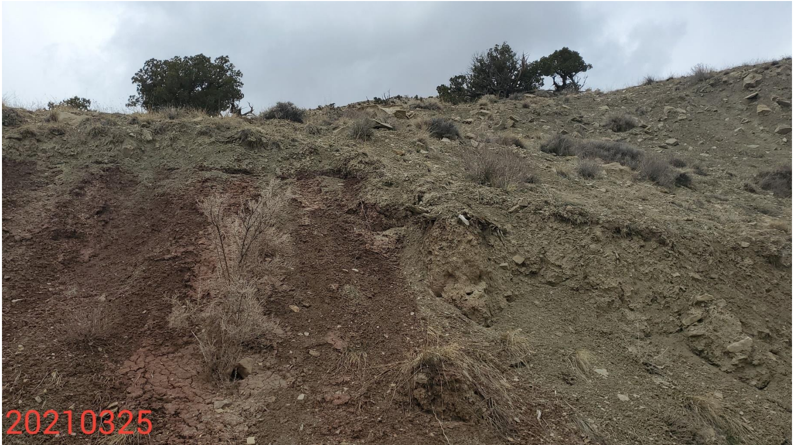
Photo 2: Photo taken from the northwest end of the Location, facing northwest. Photo shows that control measures to stabilize/protect the cut/fill slopes of the Location are missing or insufficient
