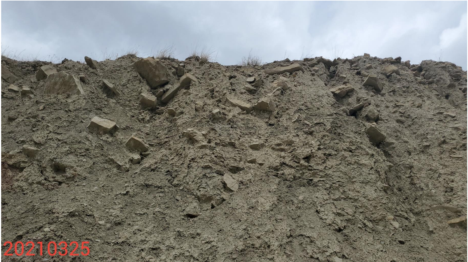
Photo 4: Photo taken from the north end of the Location, facing north. Photo shows that control measures to stabilize/protect the cut/fill slopes of the Location are missing or insufficient
