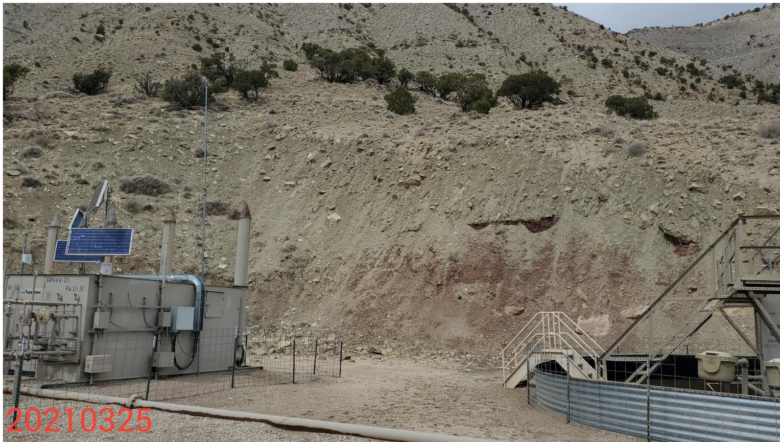
Photo 6: Photo taken from the north end of the Location, facing north. Photo shows that control measures to stabilize/protect the cut/fill slopes of the Location are missing or insufficient
