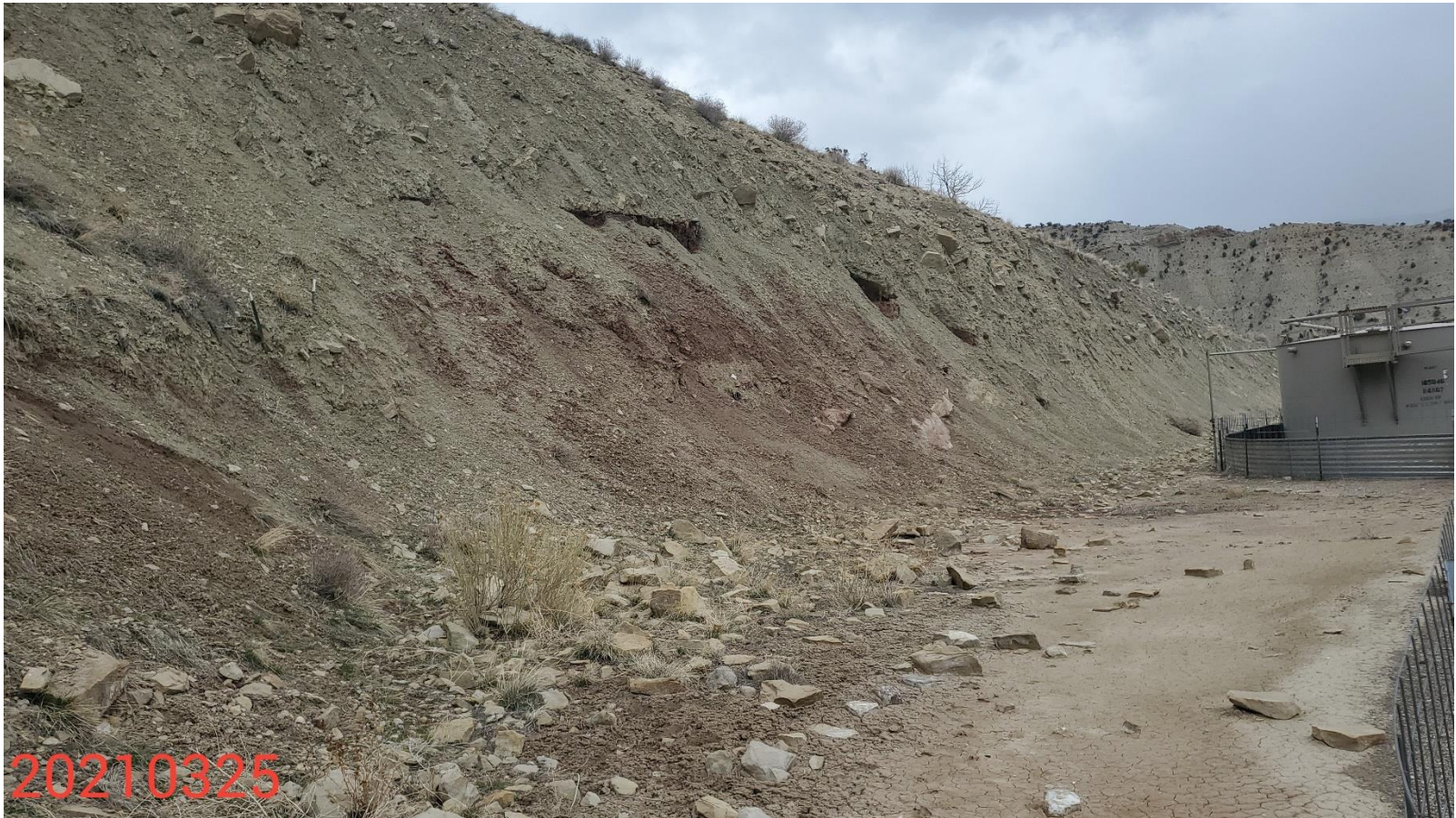
Photo 3: Photo taken from the northwest end of the Location, facing northeast. Photo shows that control measures to stabilize/protect the cut/fill slopes of the Location are missing or insufficient
