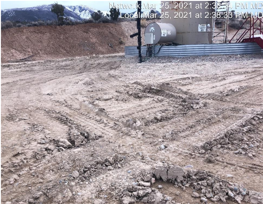
Photo #3295 Location lacks stabilization.
