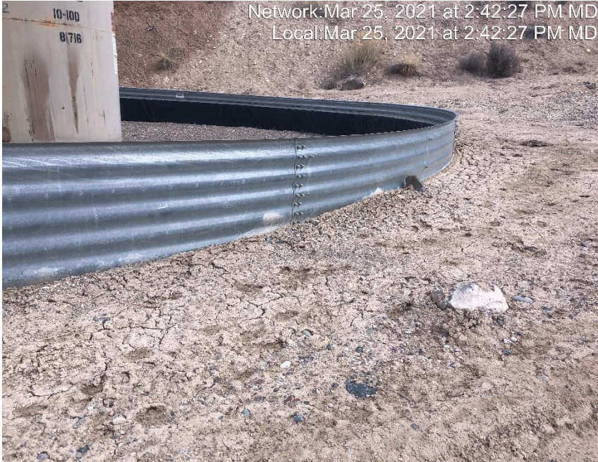
Photo #3300 Sediment has migrated on to location and is collecting against tank containment.
