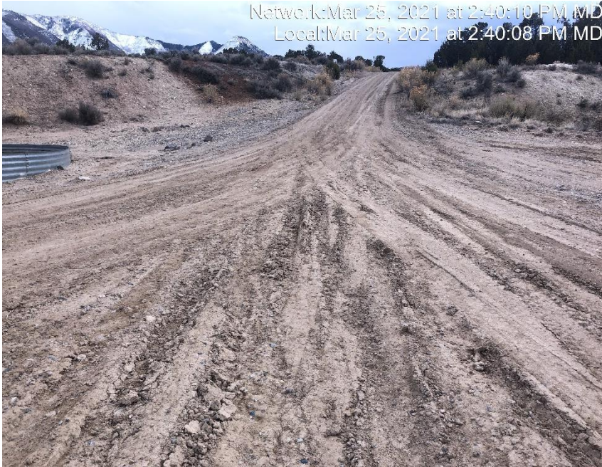
Photo #3297 No form of tracking control at entrance to location.
