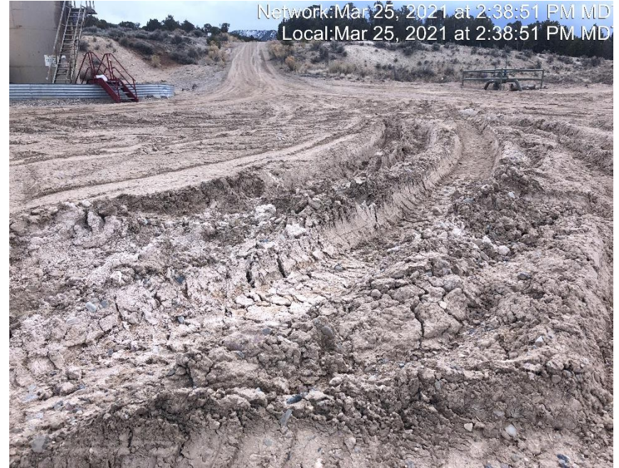
Photo #3296 Location lacks stabilization.
