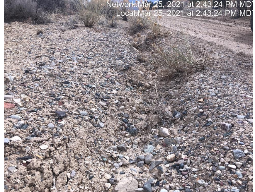
Photo #3303 Gully erosion occurring in ditch on East side of access road.
