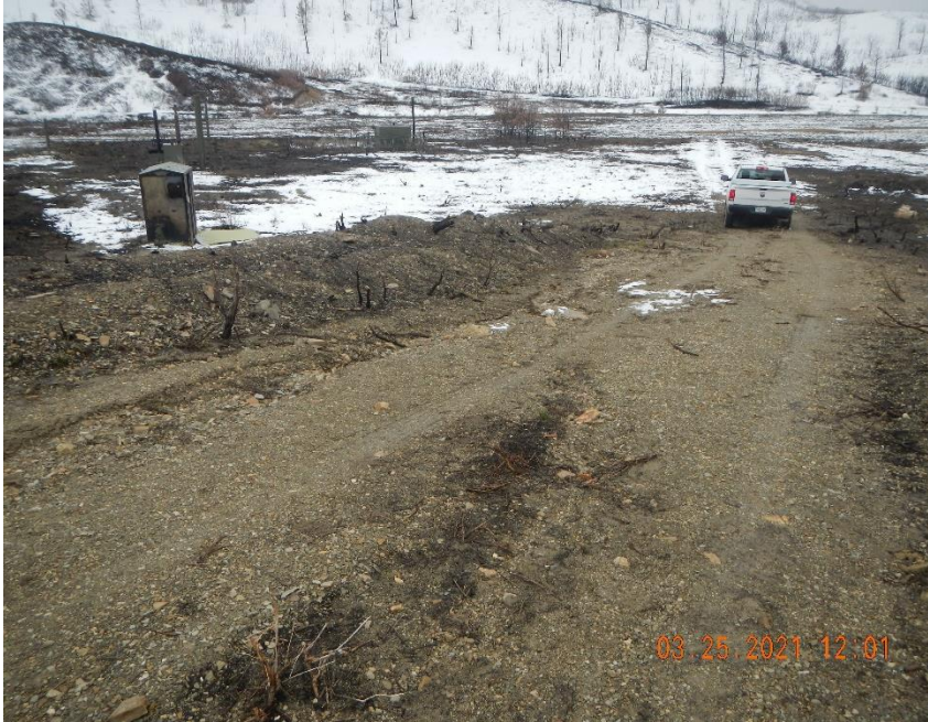
Erosion rill down roadway.
