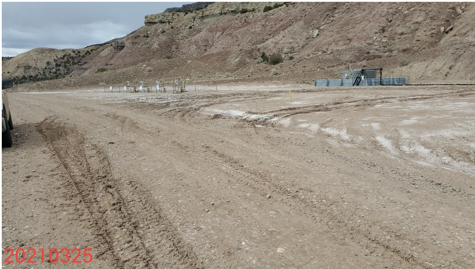
Photo 1: Photos 1-5 taken from the northern areas of the Location. Photos show that measures to stabilize/protect and minimize erosion from unpaved areas of the Location are missing or insufficient- Pad not sufficiently stabilized.
