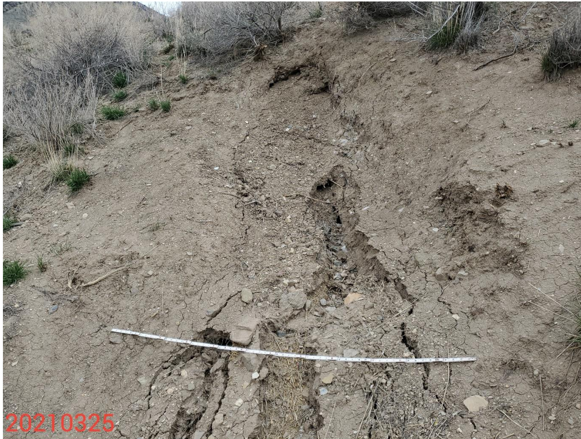
Photo 1: Photo taken from the gully erosion on slopes of the south end of the Location. Operator appears to have placed soils in an effort to repair gully, however, Operator has failed to install required stormwater and erosion control measures to stabilize and protect slopes. 6 foot measuring stick for reference.
