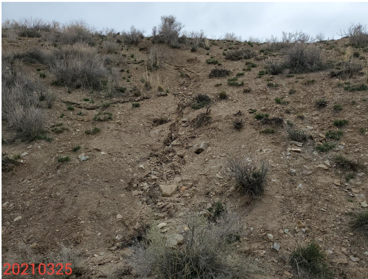
Photo 4: Photo taken from the gully erosion on slopes of the south end of the Location. Operator appears to have placed soils in an effort to repair gully, however, Operator has failed to install required stormwater and erosion control measures to stabilize and protect slopes. 6 foot measuring stick for reference.
