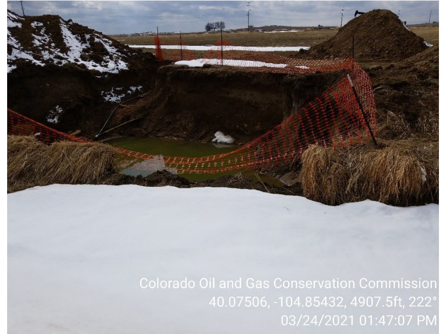
Photo 2 – Collapsed wall of Brantner Irrigation ditch into open excavation.
