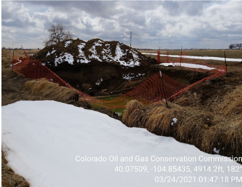
Photo 1 – Open spill excavation adjacent to Brantner Irrigation ditch. A portion of the irrigation ditch wall has collapsed into open excavation; remaining portion of the ditch wall next to excavation appears unstable.
