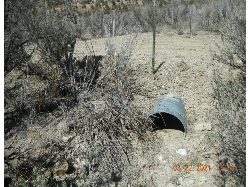
Culvert outlet partially packed with sediment.
