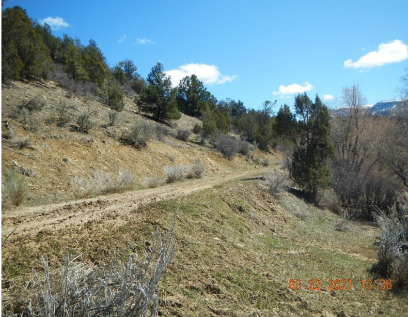
Sediment moving over shoulder of access road.
