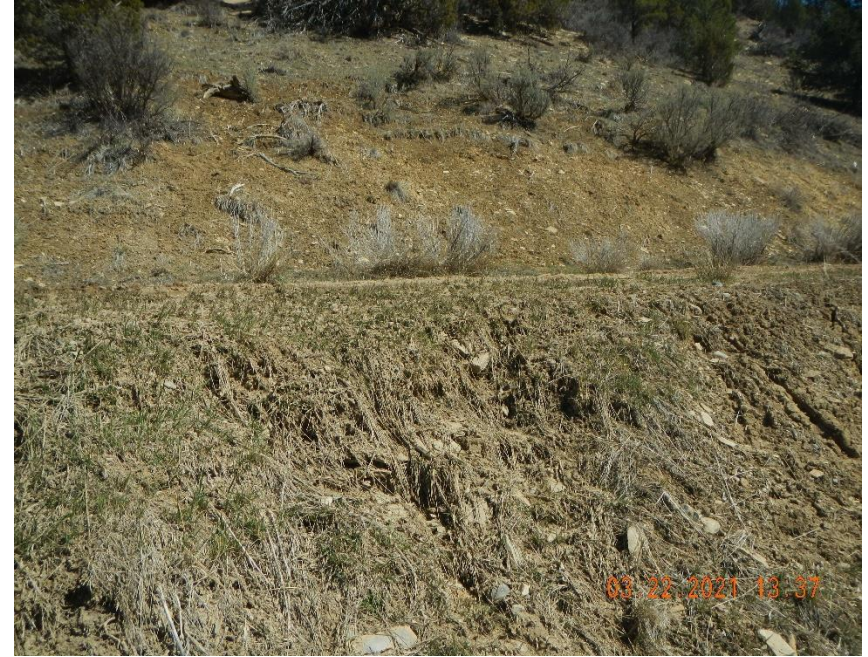
Washing erosion of road embankment.
