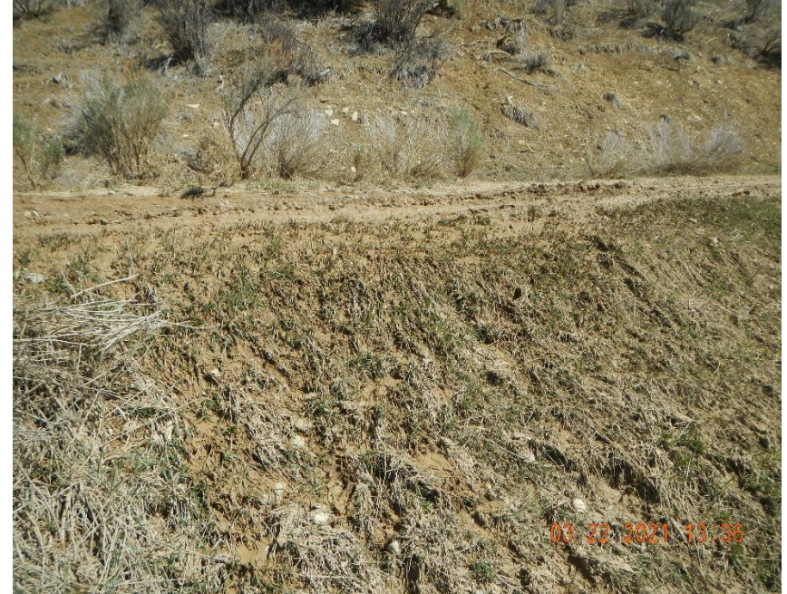
Sediment moving over shoulder of access road.
