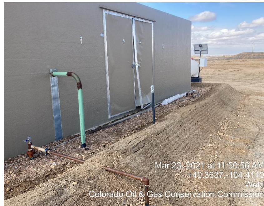
Photo #4 Repaired Berm
