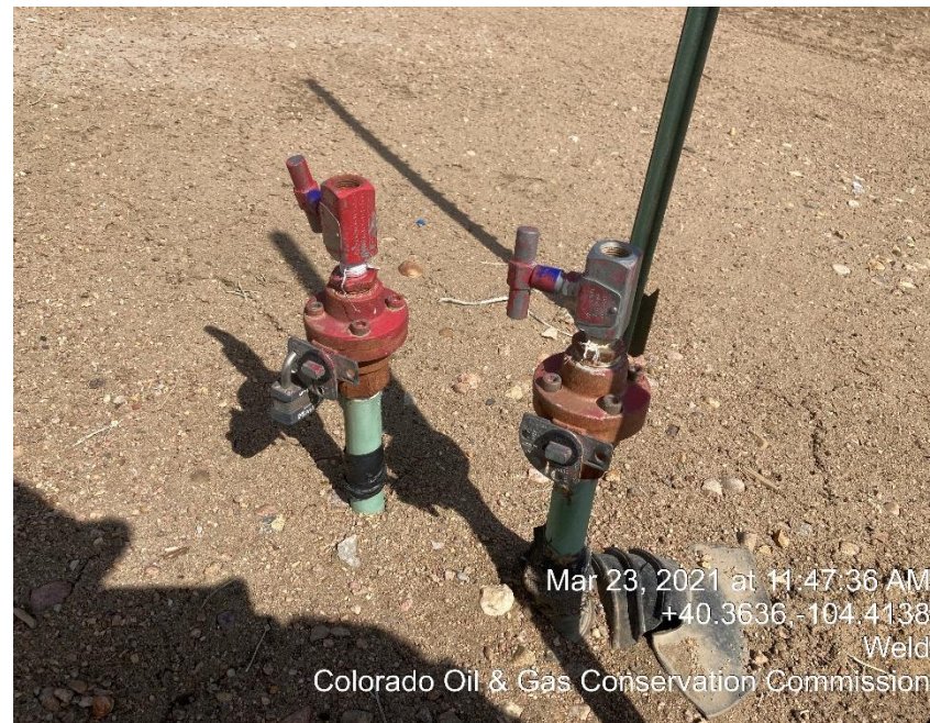
Photo #8 Not "LO/TO" or Marked on both risers
