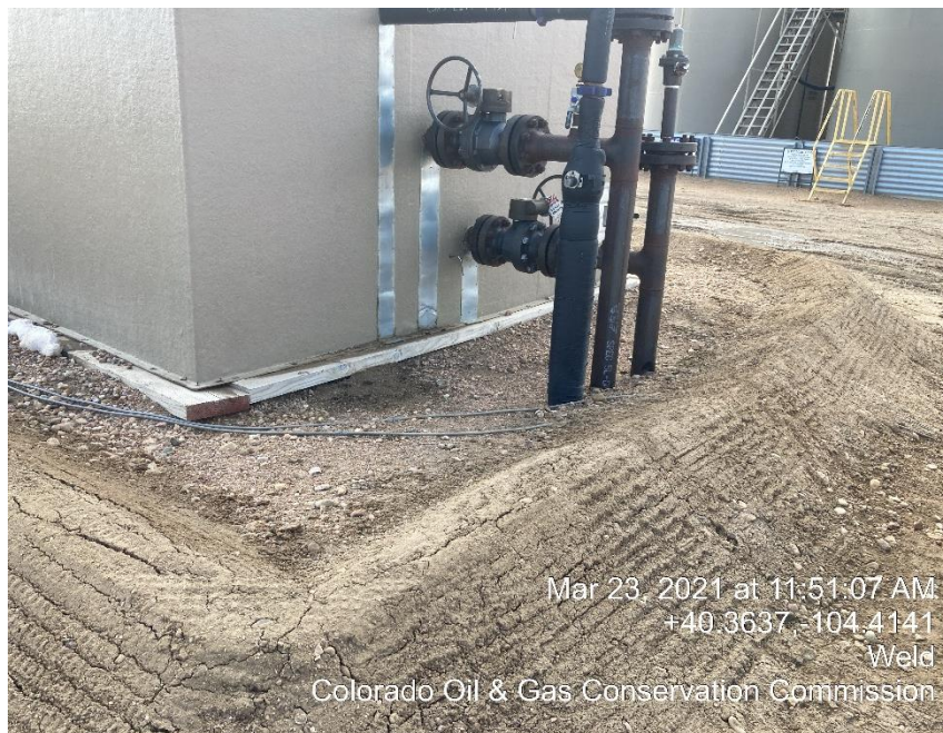
Photo #5 Repaired Berm
