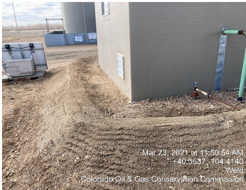
Photo #3 Repaired Berm
