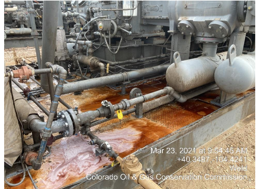
Photo #10 Oily Skid/ Mechanical Conditions
