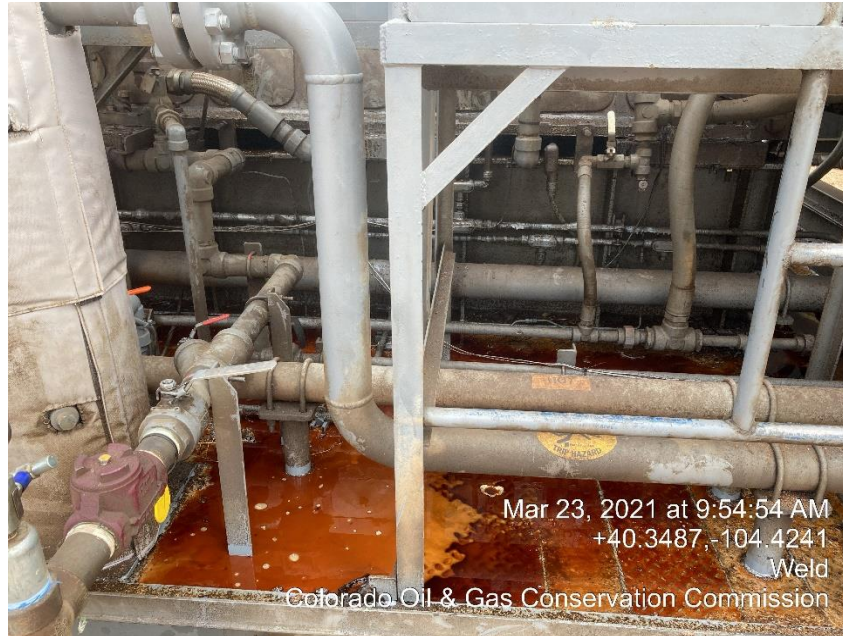
Photo #11 Oily Skid/ Mechanical Conditions
