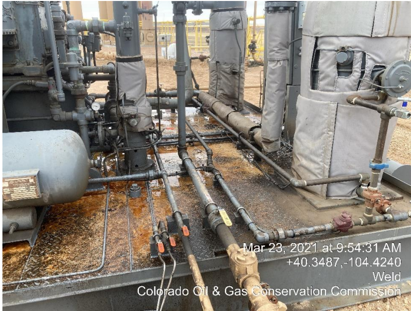
Photo #9 Oily Skid/ Mechanical Conditions
