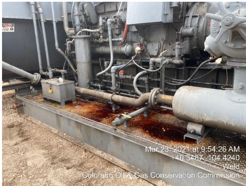
Photo #7 Oily Skid/ Mechanical Conditions
