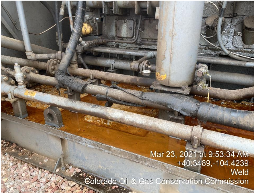
Photo #3 Oily Skid/ Mechanical Conditions
