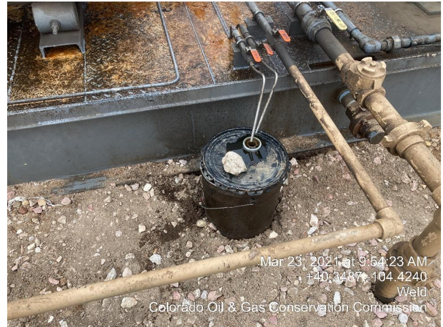
Photo #13 Packing vent lines dripping into bucket
