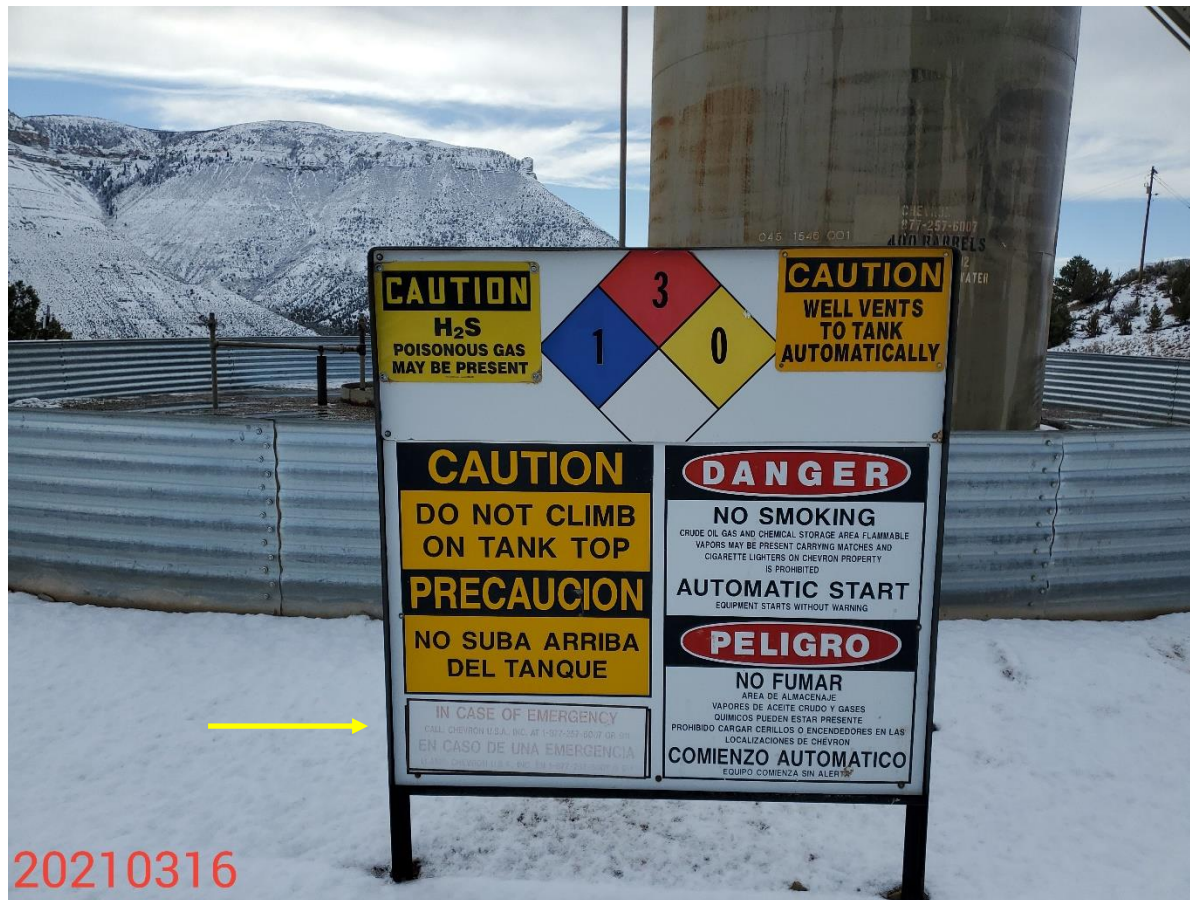
Photo 9: Photo of signage at the tank. Photo shows the emergency contact label on the sign is fading, and becoming difficult to read. Maintenance advised.
