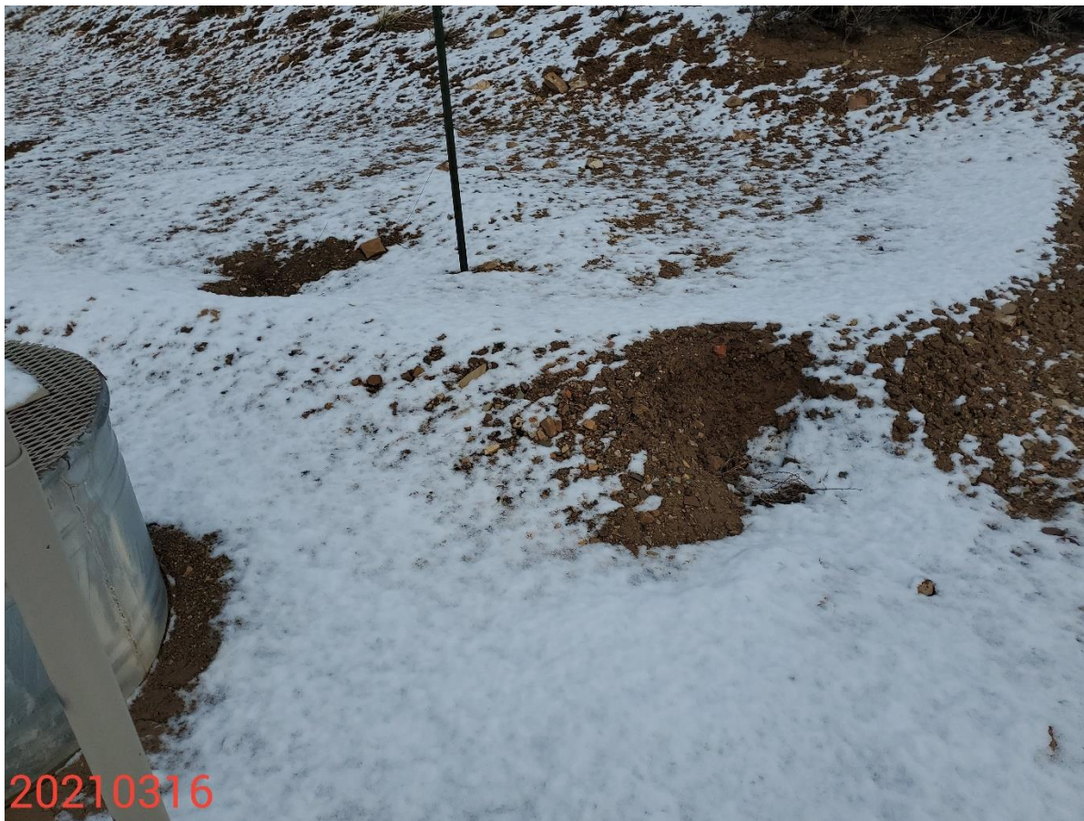
Photo 11: Photo taken from containment berm around the separator equipment on the northeast end of the Location. Wildlife appear to be digging into the containment BMP; Ensure integrity of the containment BMP remains adequate.
