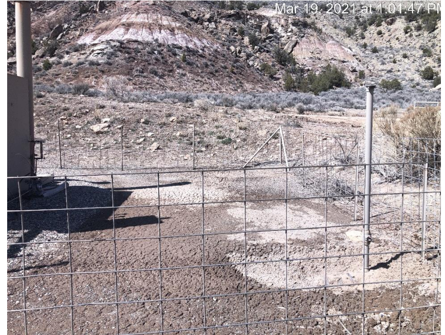
Sediment build up in back corner of fence.
