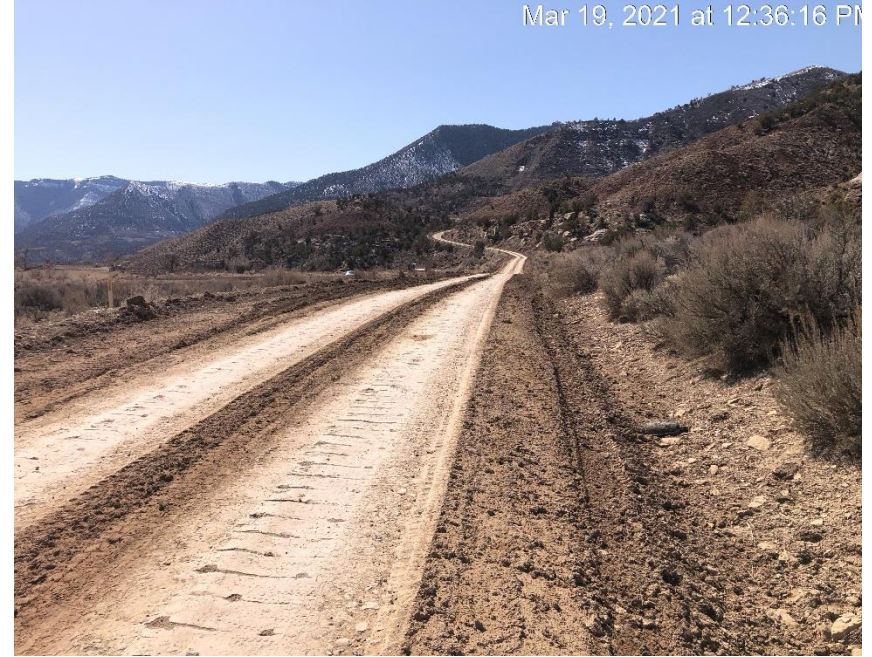
Ditch damaged from traffic.
