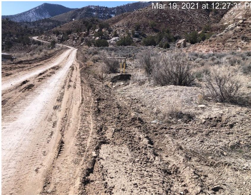
Sediment build up and traffic damage in ditch.
