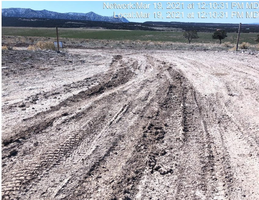
Photo #3207 No form of tracking control at entrance to location.
