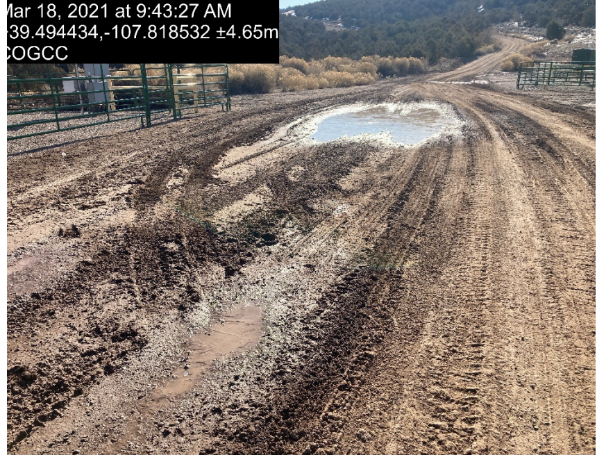
location entrance/Lack of stabilization/compaction
