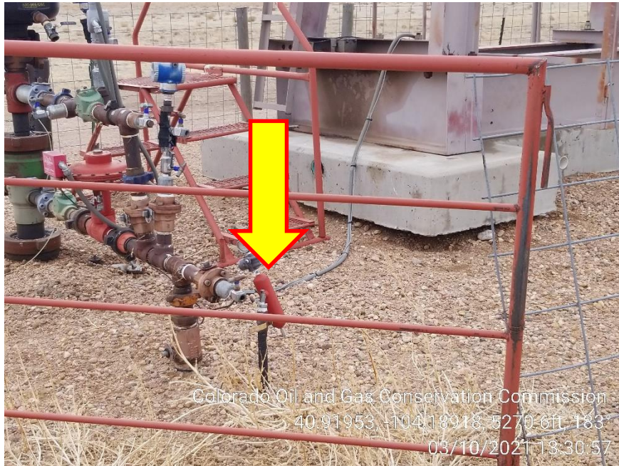
Photo 3 – Unmarked 1" Riser at Wellhead
