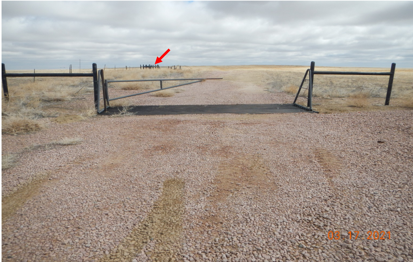
Photo 1. Facing north at the beginning of the access road. The gravel and cattleguard remains and the fence has not been put back to original place. Additional H-brace posts are shown at red arrow.
