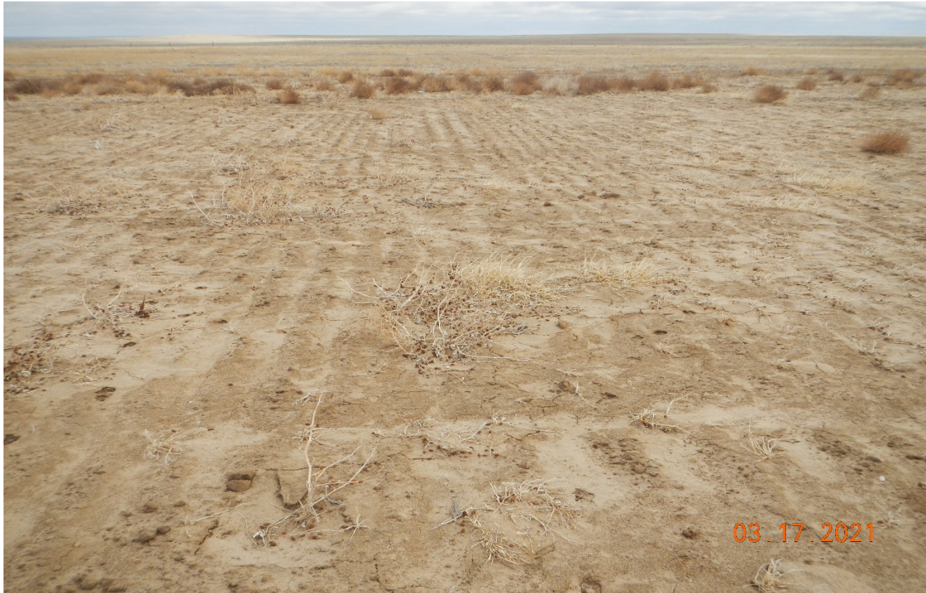
Photo 3. Facing south towards the location. It appears the location has been cross-ripped. The location needs to be seeded and stabilized.
