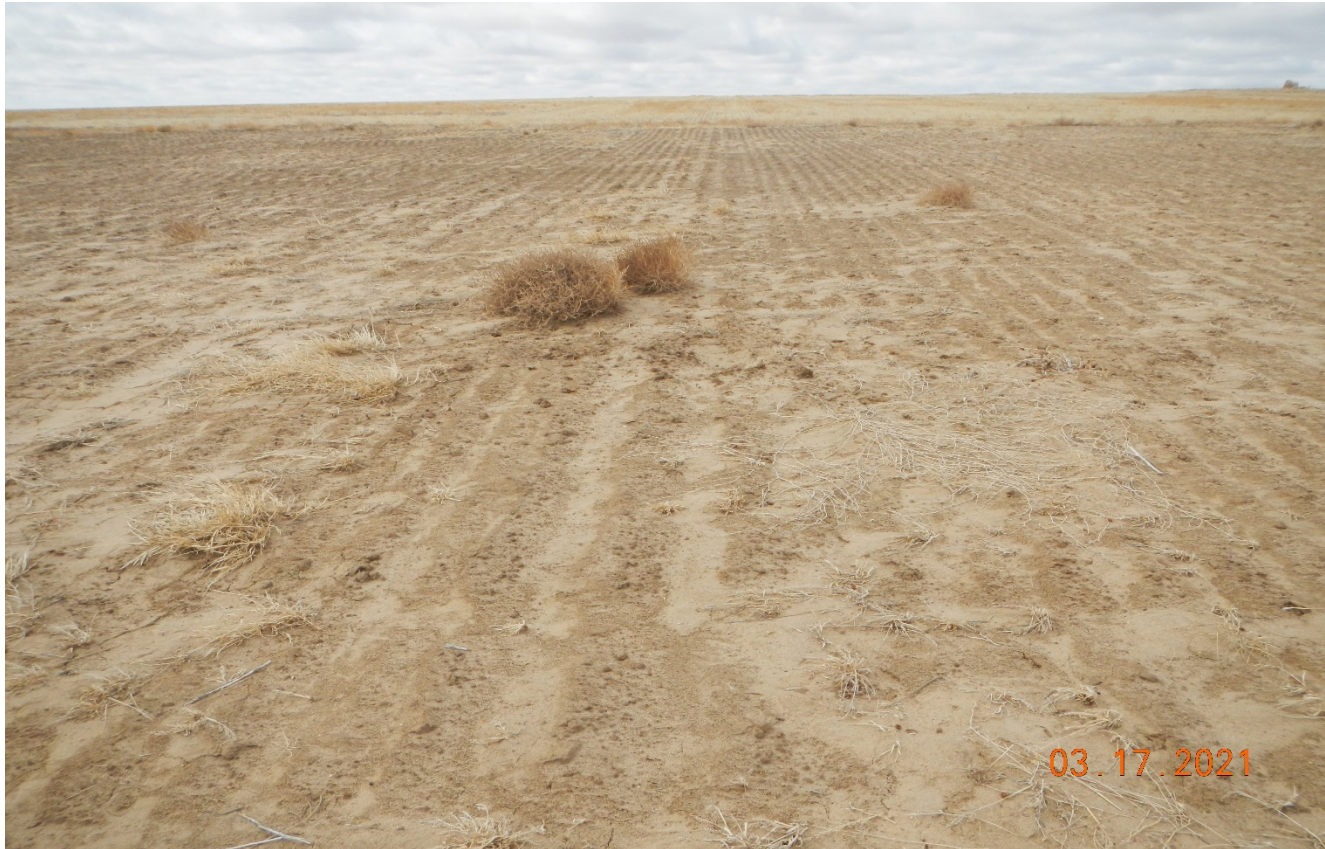
Photo 4. Facing west towards the location. It appears the location has been cross-rippled. The location needs to be seeded and stabilized.
