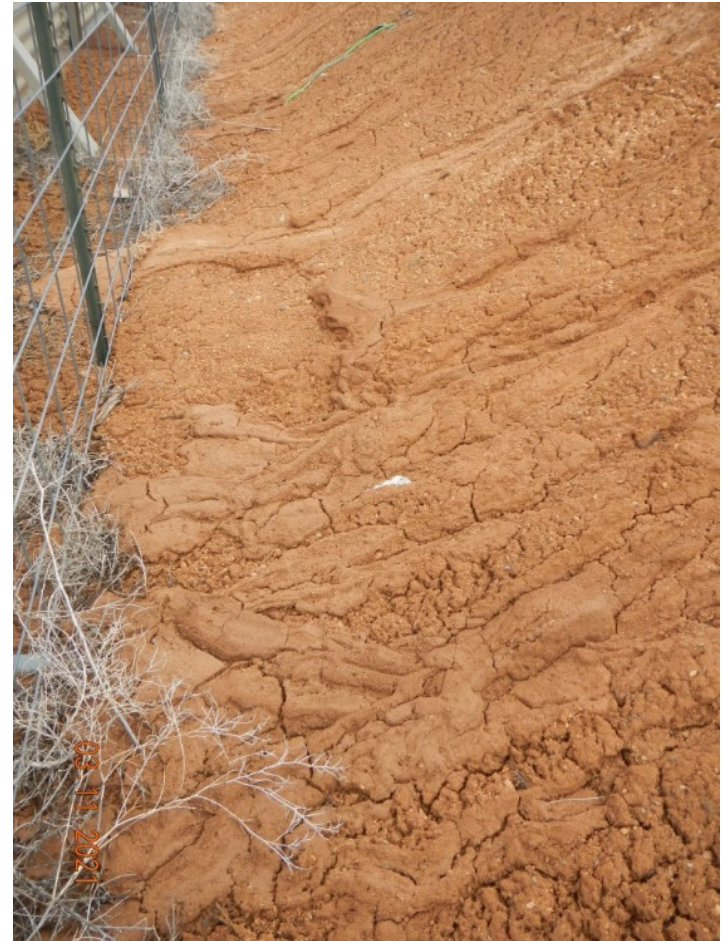
Photo#3: Erosion, sediment migration on Cut.
