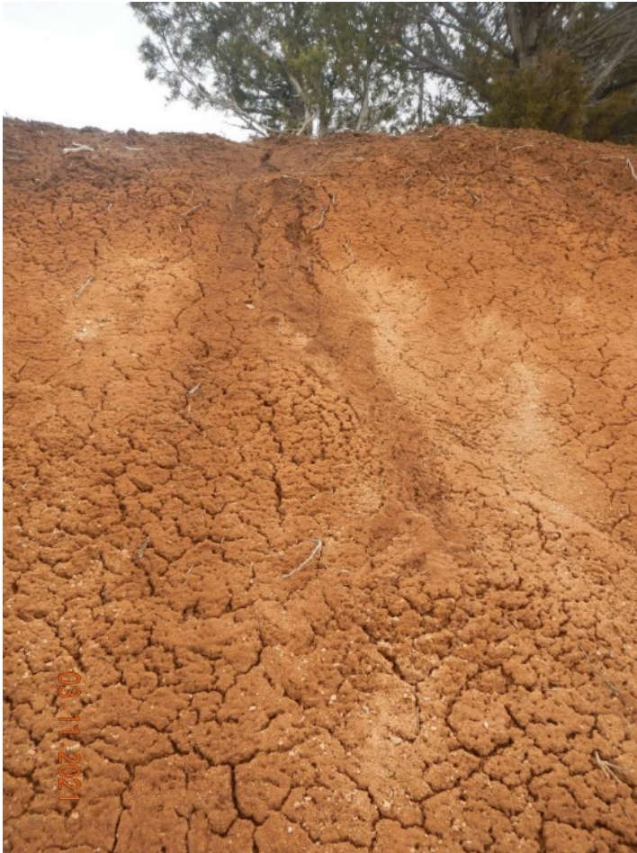
Photo#2: Erosion, sediment migration on Cut.
