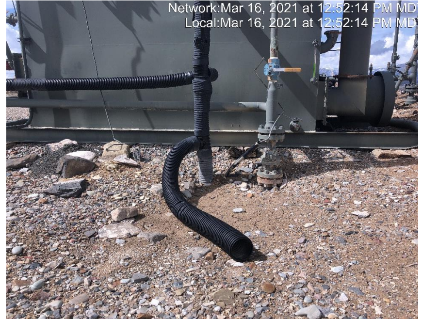
Photo #3155 Flow line heating insulation open ended and not capped.
