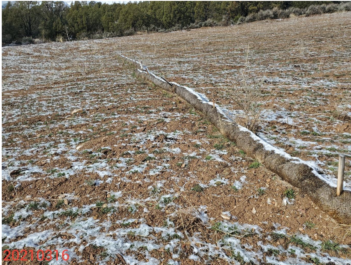
Photo 1: Photo taken from the Location. Photo shows example of wattles on the Location; it was observed that wattles have not been installed in accordance with good engineering practices (trenched and backfilled).
