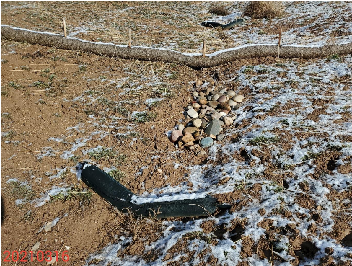
Photo 2: Photo taken from the southern area of the Location where channelized erosion has been documented. Photo shows Operator has placed rock aggregate, as well as rock socks within the area of erosion. Photo also shows wattle BMPs on the Location remain improperly installed.
