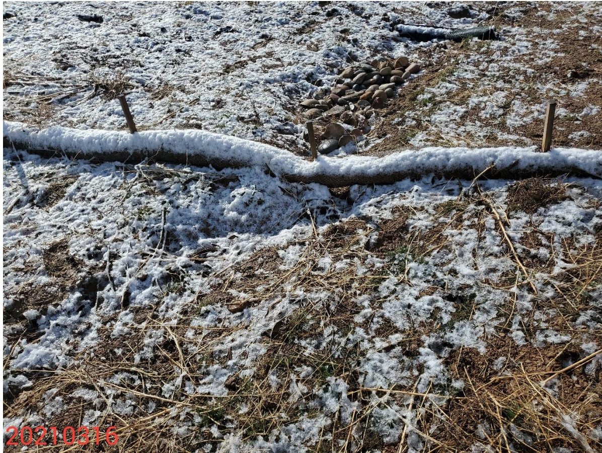
Photo 3: Continued from photo 2. Photo shows wattles on the Location have not been installed in accordance with good engineering practices (trenched and backfilled).
