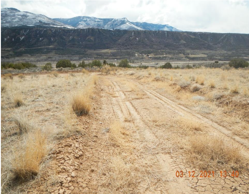
Weed debris on access road into location. Access road lacks stabilization.
