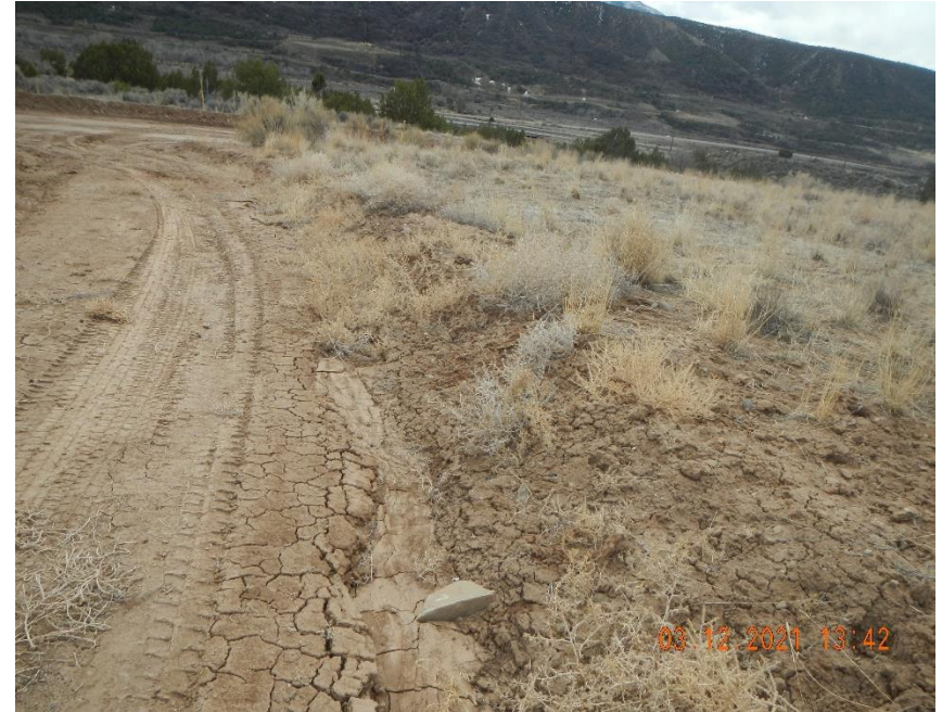
Ditch on access road needs maintained.
