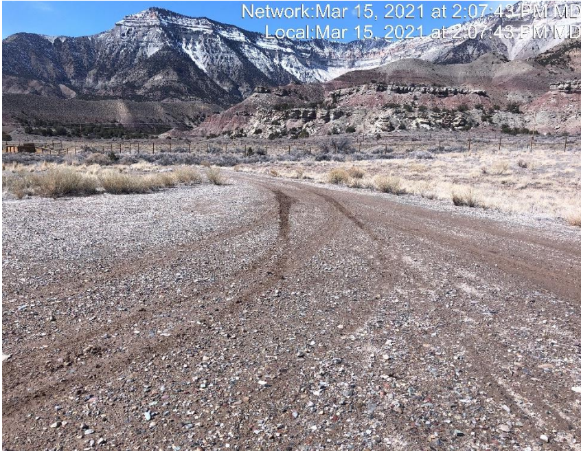
Photo #3152 No form of tracking control at entrance to location.
