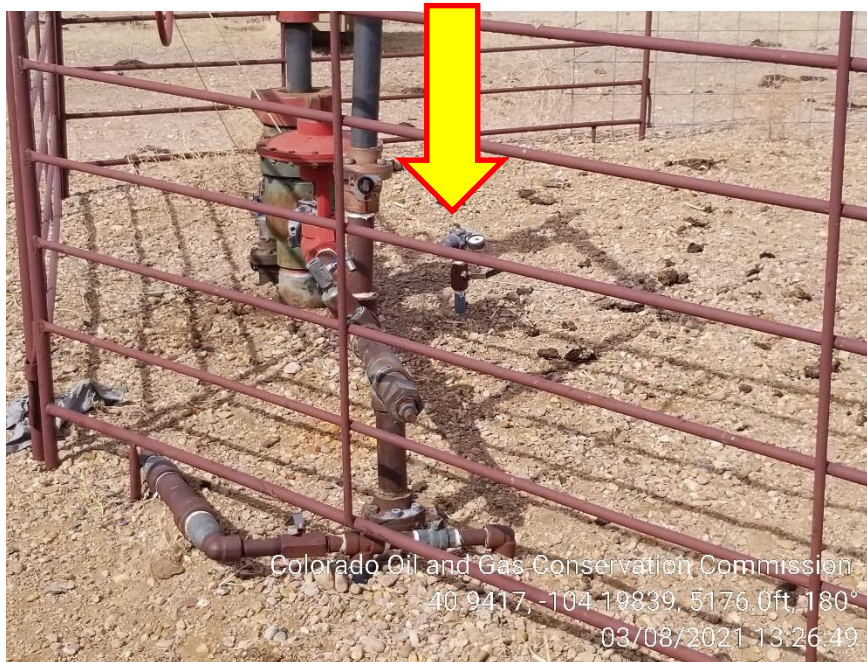
Photo 3 – Unmarked 1" Riser
