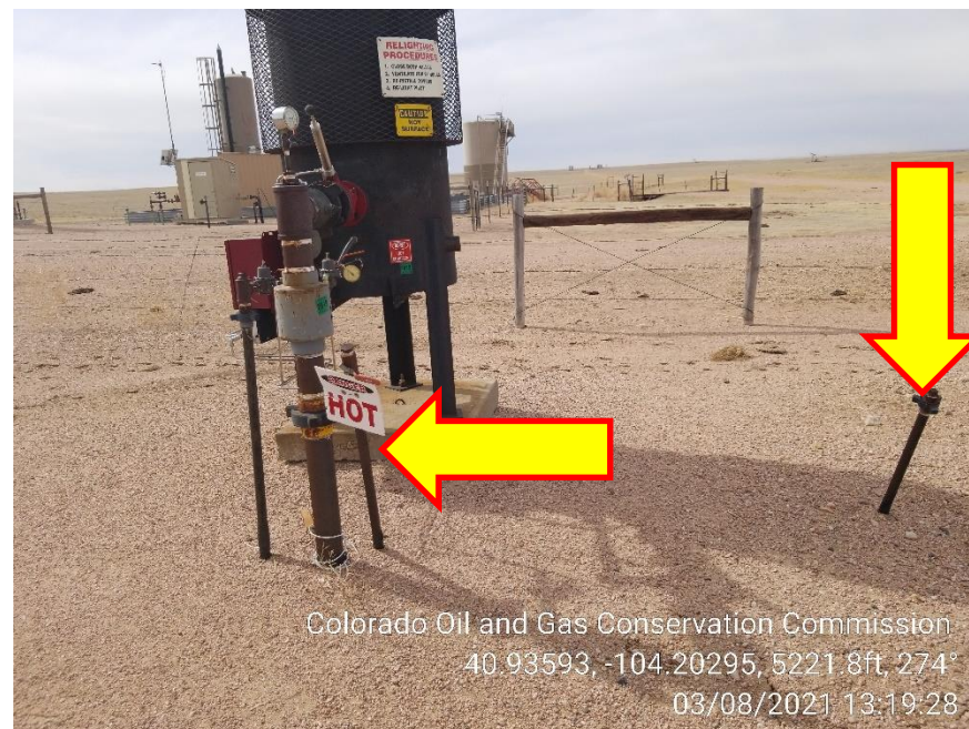
Photo 4 – Unmarked 1" Risers at ECD
