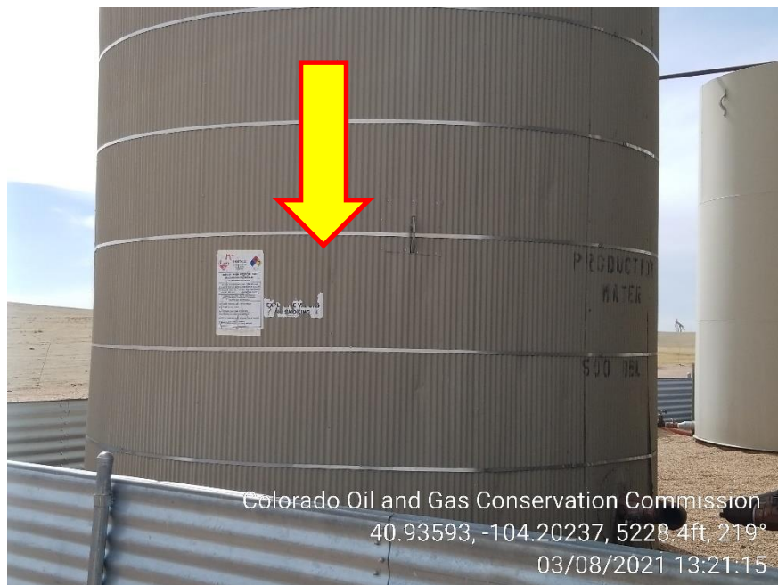
Photo 3 – 500 H2O Tank missing NFPA Label
