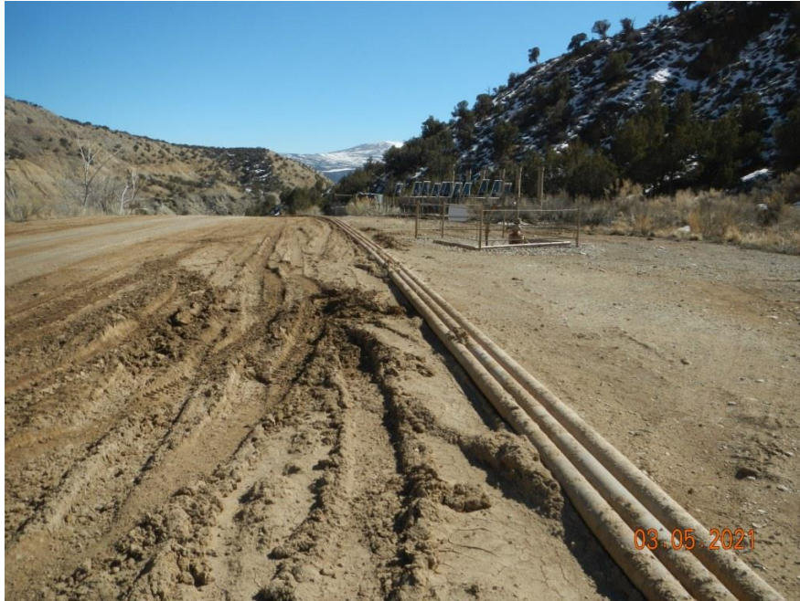
Photo#2: Rutting, degradation of site.
