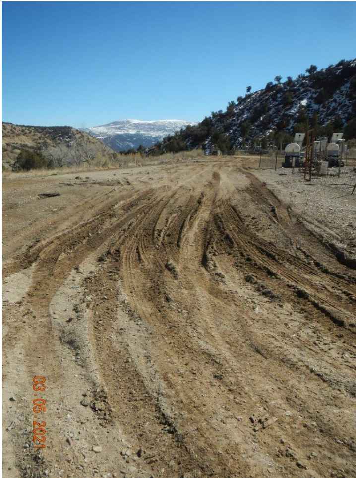
Photo#3: Rutting, degradation of site.
