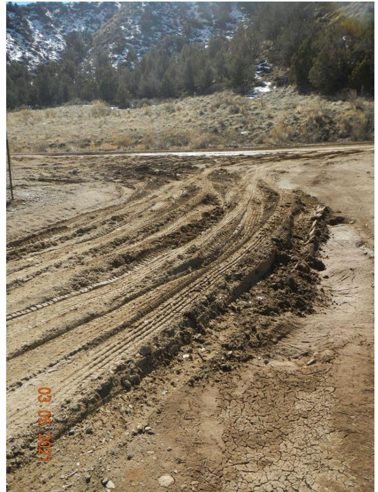
Photo#4: Rutting, degradation of site.
