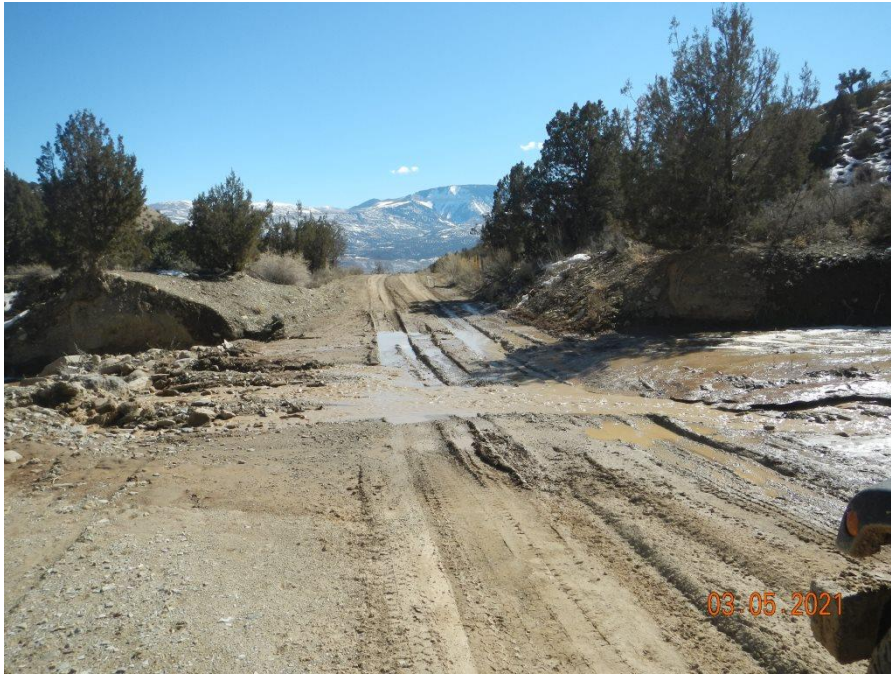
Photo#2: Stream crossing needs maintenance/stabilization.
