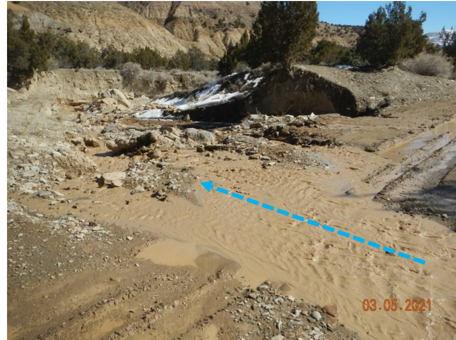
Photo#3: Stream crossing needs maintenance/stabilization, view to East with flow.
