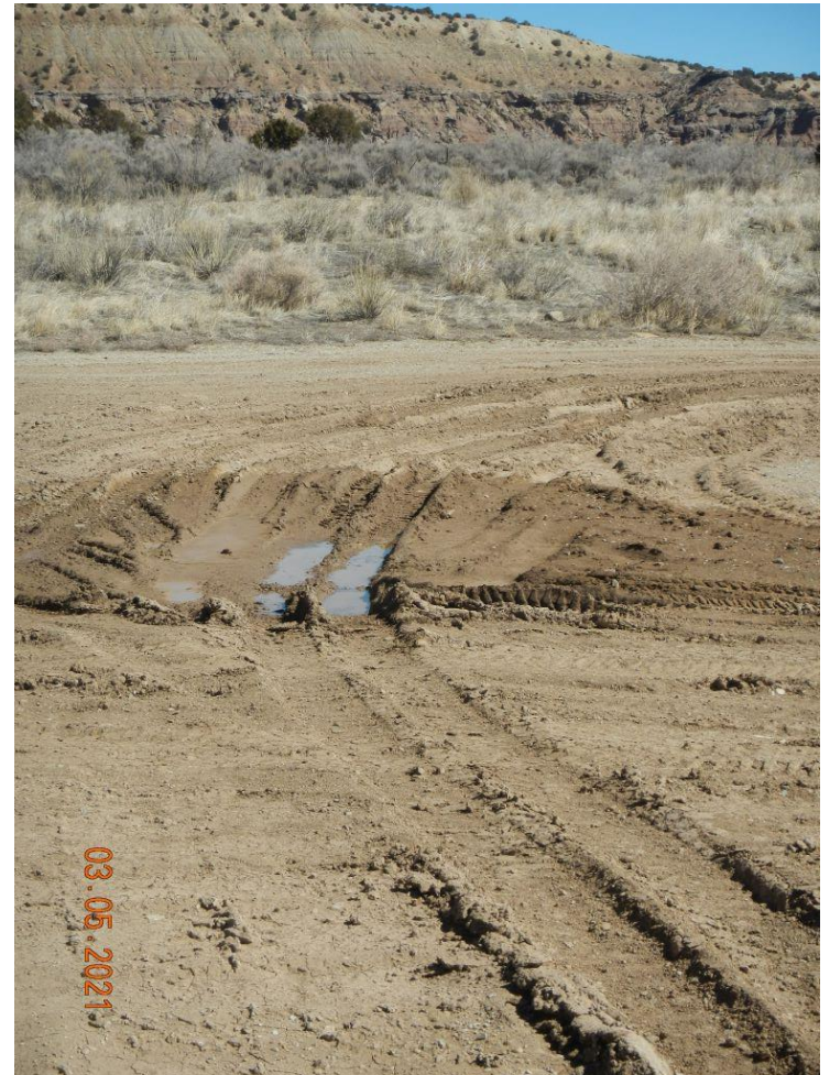
Photo#3: Rutting at entry to location..
