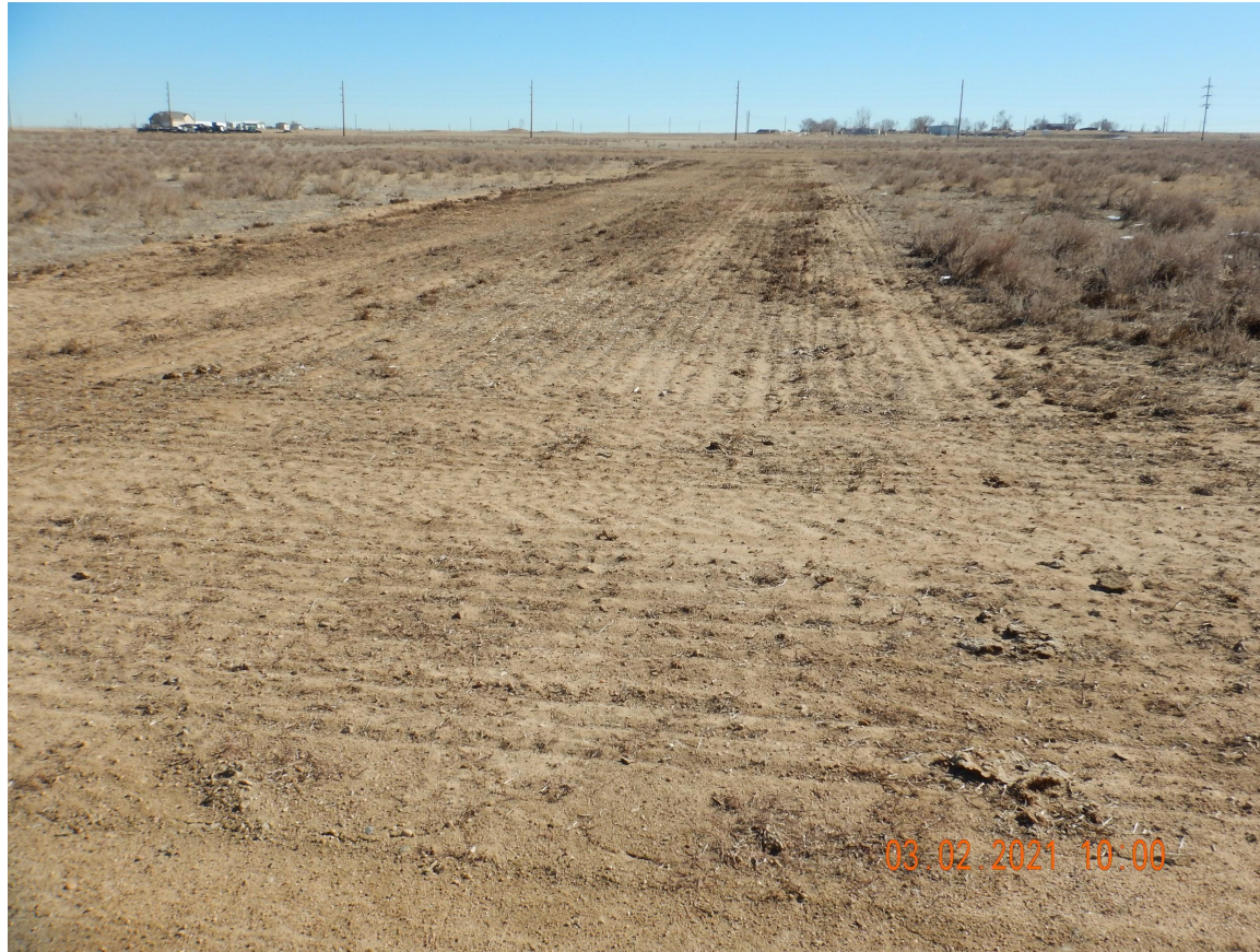
Photo 2. Photo taken from the western well location access road, facing East. Photo illustrates Operator has performed final reclamation activities (i.e., seeding) with the evidence of drill rows.
