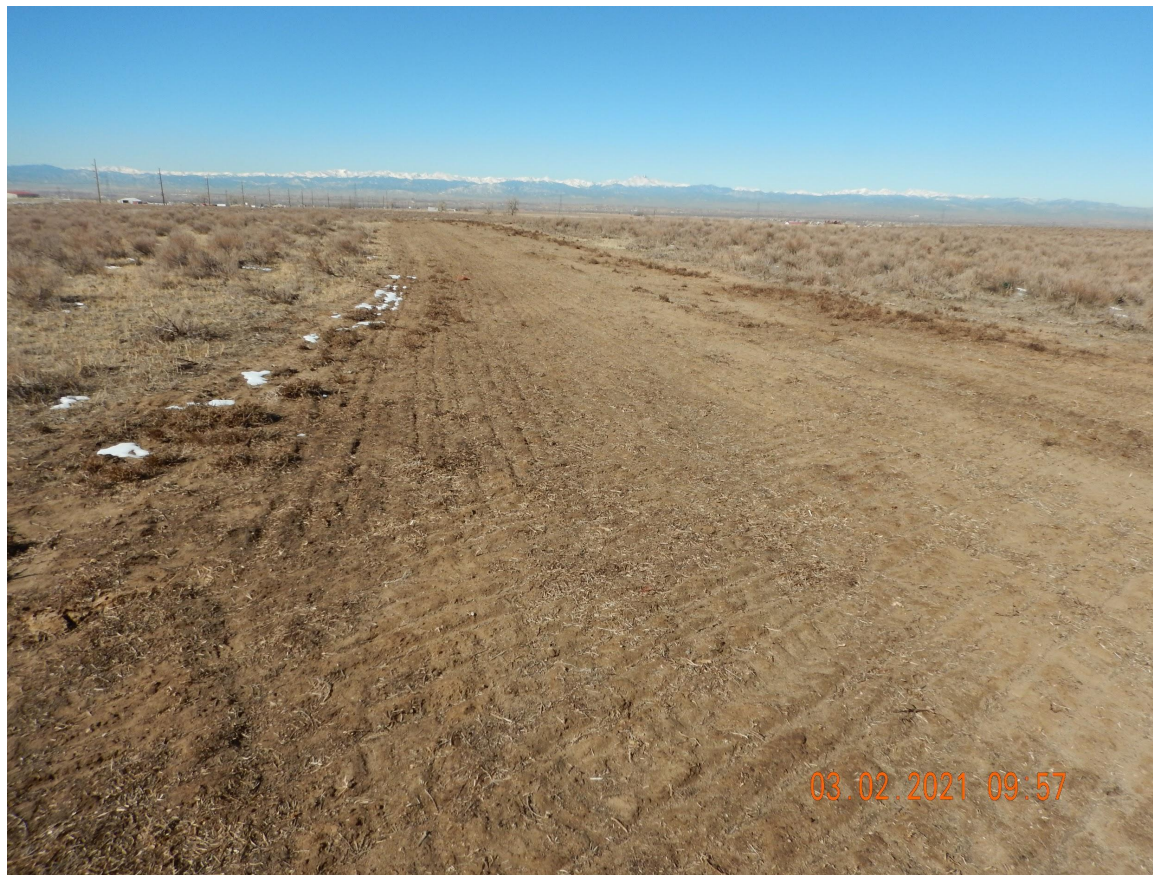
Photo 2. Photo taken from the eastern well location access road, facing West. Photo illustrates Operator has performed final reclamation activities (i.e., seeding) with the evidence of drill rows.
