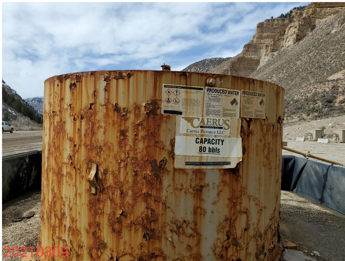
Photo 6: Photo of 80 bbl tank on Location. Signage peeling off. Inspection #701100324 observed that the tank is rusted and peeling paint. Inspection required Operator to "Inspect, maintain and repair tanks following standard industry practice such as API 12R" by 11/3/2020. Corrective action from FIR 701100324 does not appear to have been addressed.
