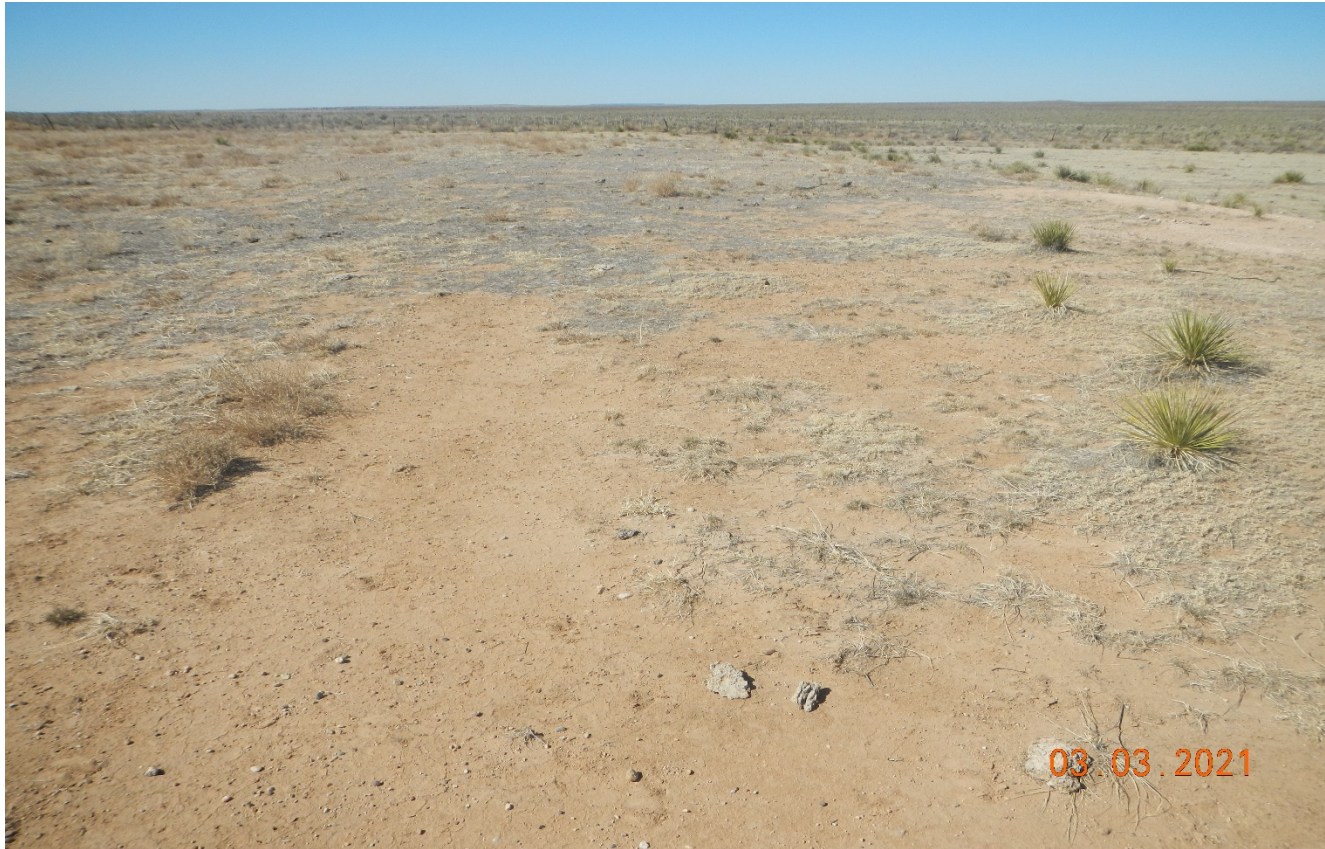
Photo 5. Facing west at the northeast side of the location. The fill slope has not been recontoured. The area along the fill slope is compacted and should be leveled to match the contours of the terrain.
