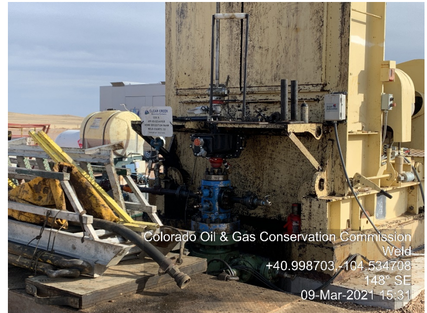
Photo #2 Cox 5 (05-123-41935) Wellsite Shut-In | SI Workover completed. Had parted rods.
