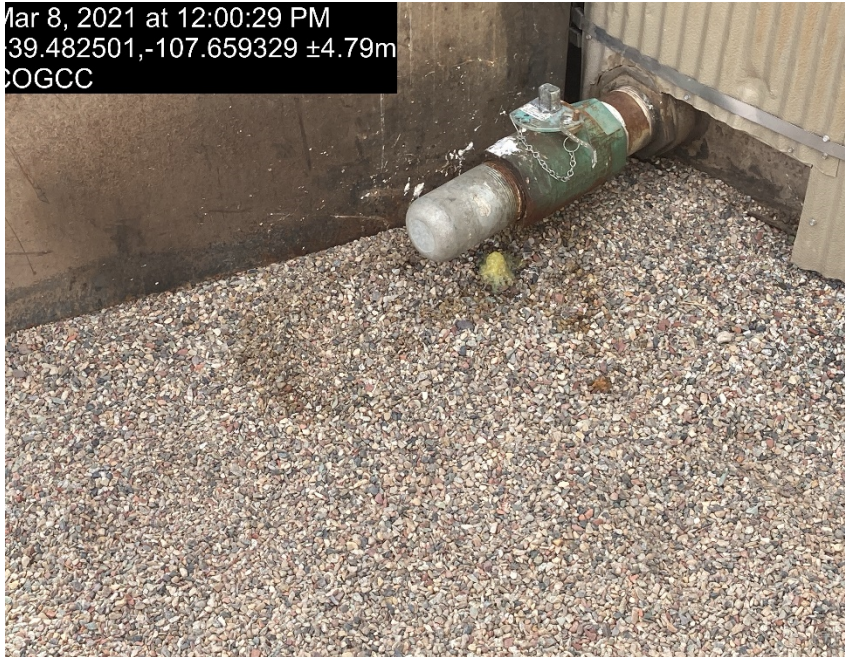
Staining/valve leaking
