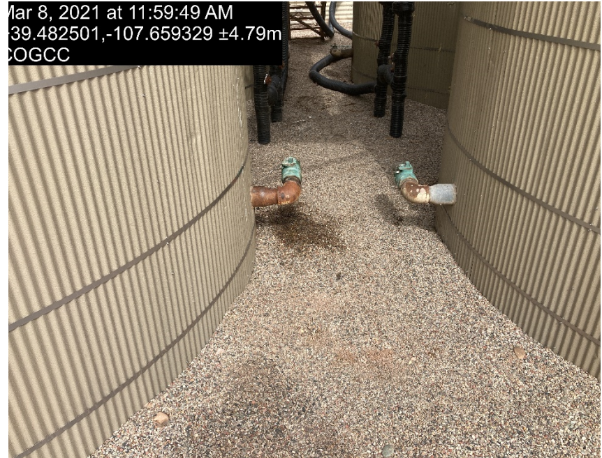
Staining/valve leaking
