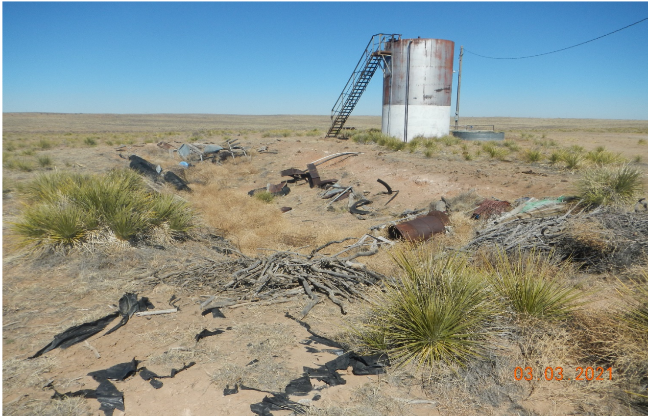
Photo 4. Facing northeast toward the pit. The pit liner is torn and degraded. There is various debris in the pit. The pit was never closed and reclaimed as required.
