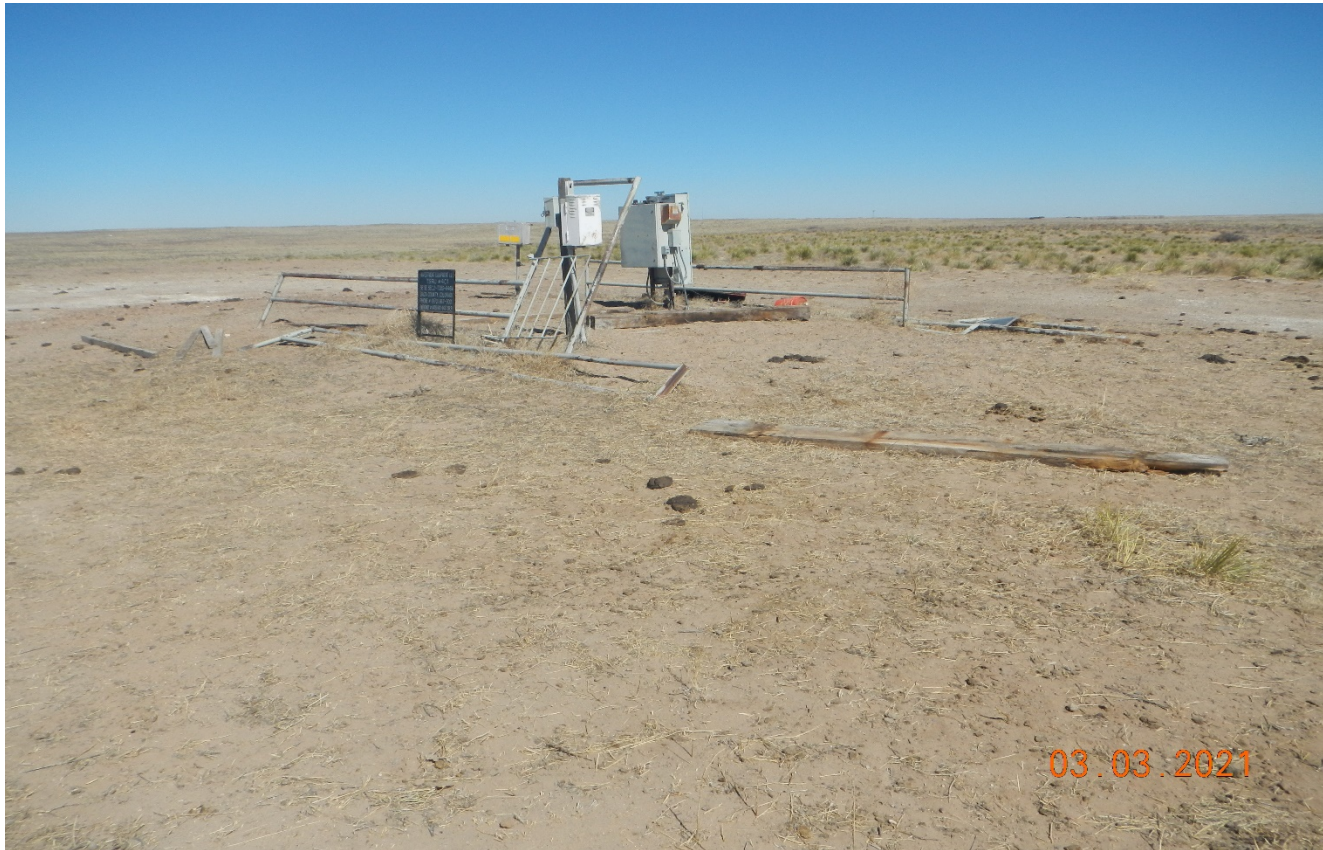
Photo 1. Facing northeast toward the well site. The location has not been reclaimed. Equipment and debris remains at the location. All equipment should have been removed within 3 months of abandoning the well.
