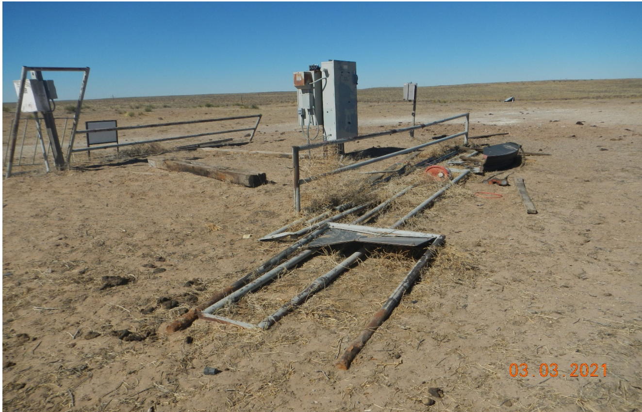
Photo 2. Equipment and debris remains at the location. All equipment should have been removed within 3 months of abandoning the well.
