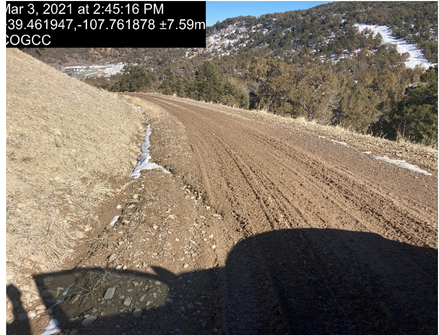
Lease road/Access road lack of compaction
