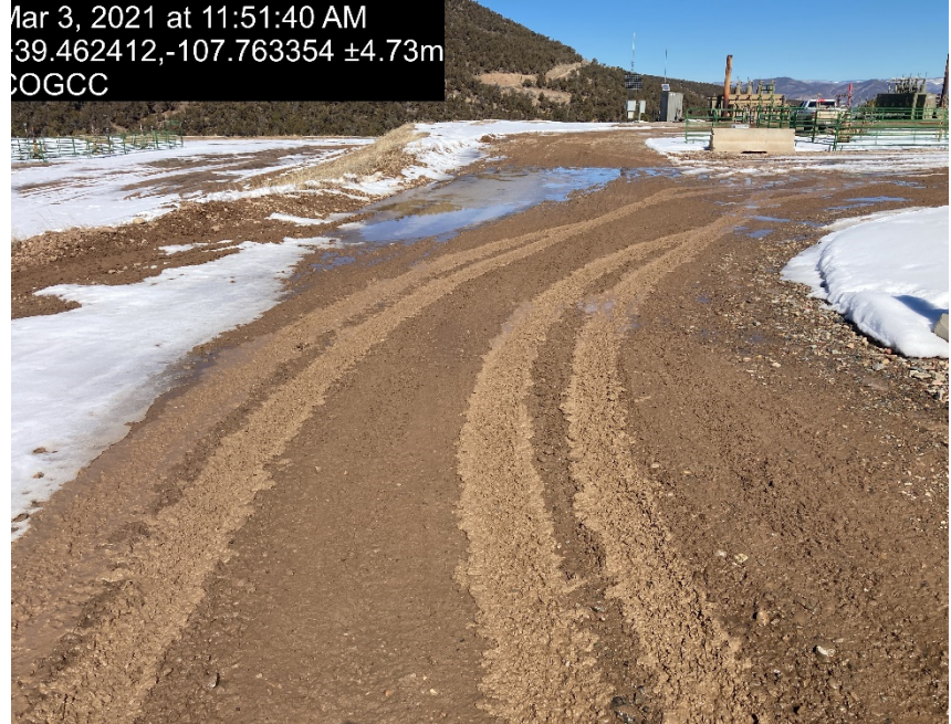
location/entrance/lack of compaction
