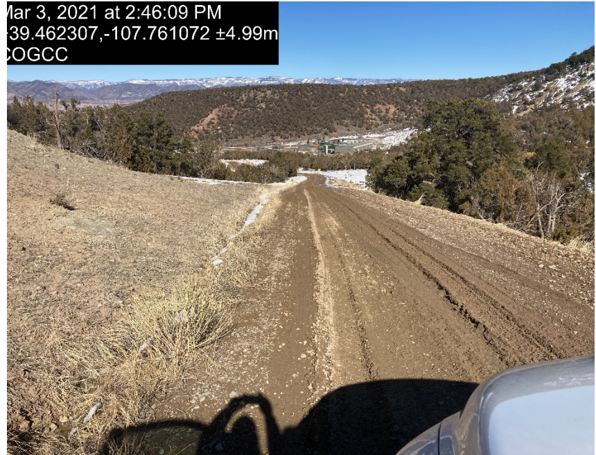
Lease road/Access road lack of compaction
