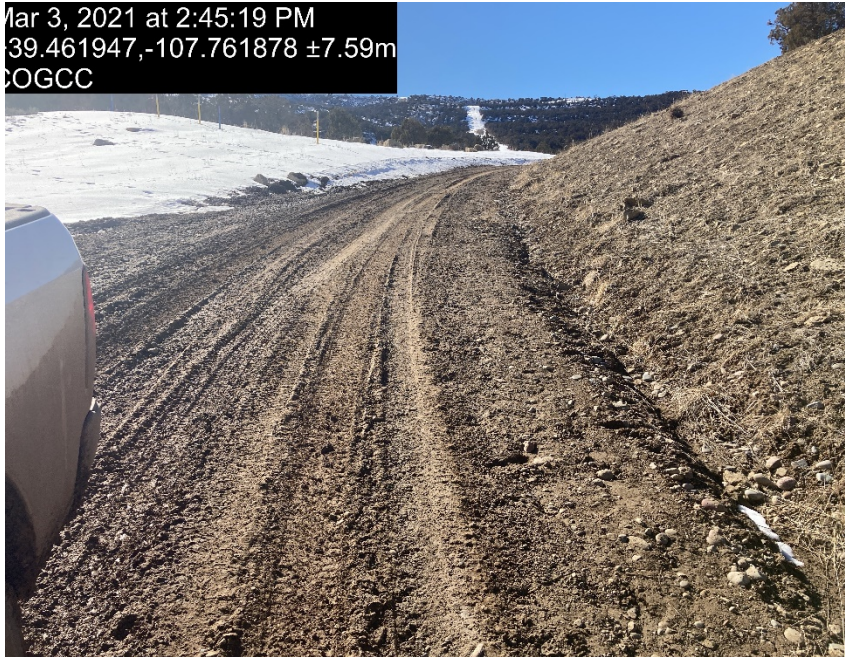
Lease road/Access road lack of compaction
