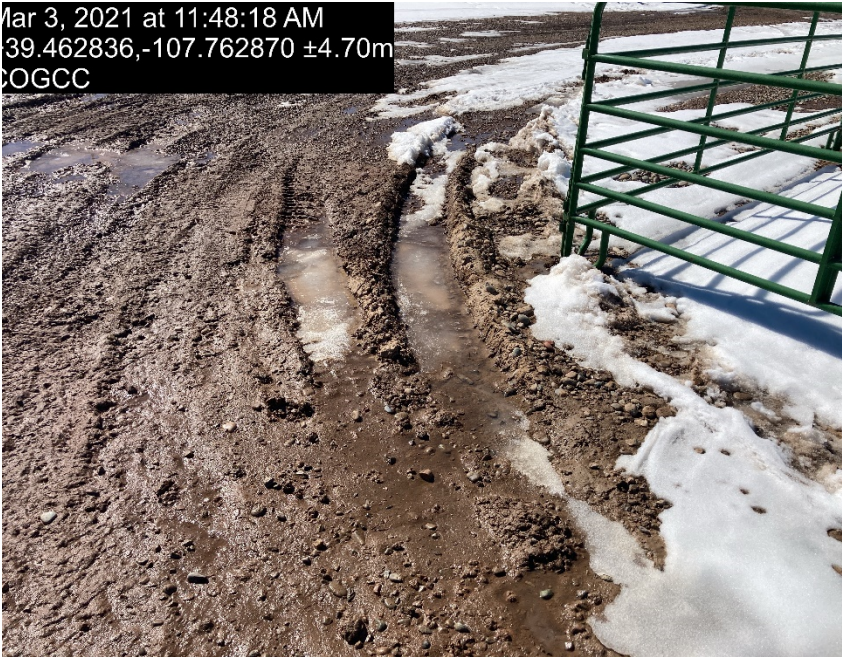
lack of compaction/stabilization
