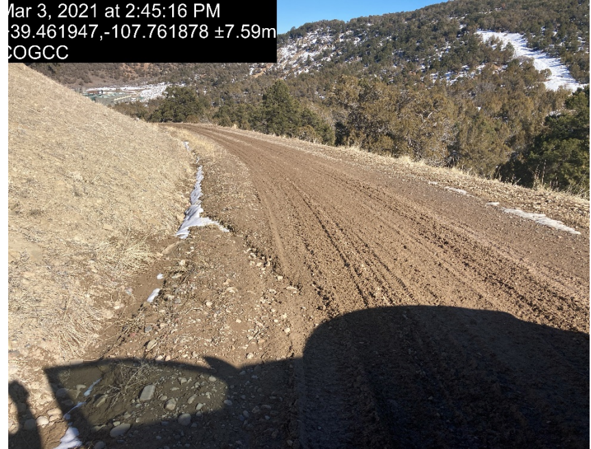
Lease road/Access road lack of compaction
