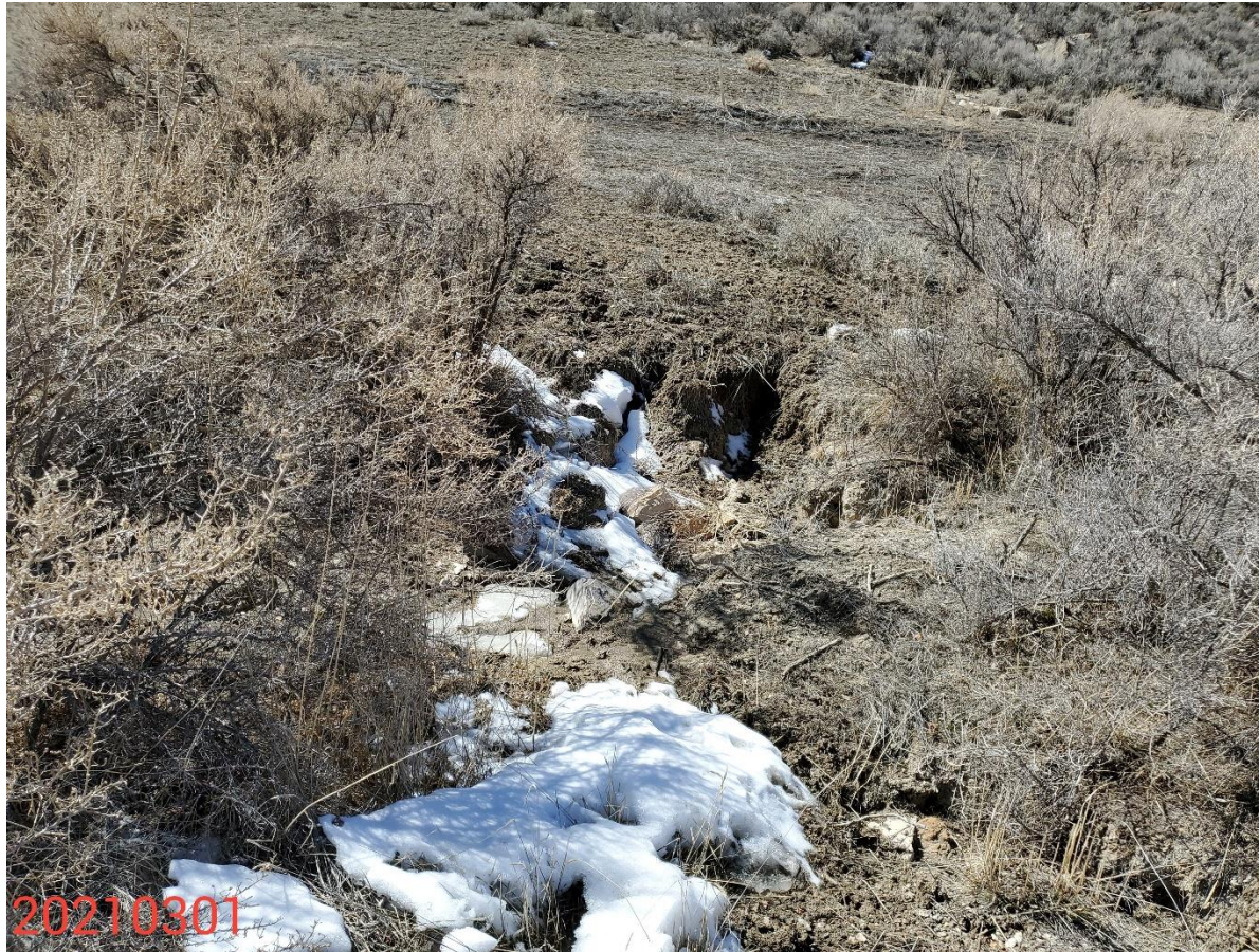
Photo 16: Photo taken from below the sediment trap outlet observed in photo 15. Photo shows areas below the sediment trap outlet where head cutting and gully erosion degradation due to runoff is occurring. Control measures missing or insufficient.
