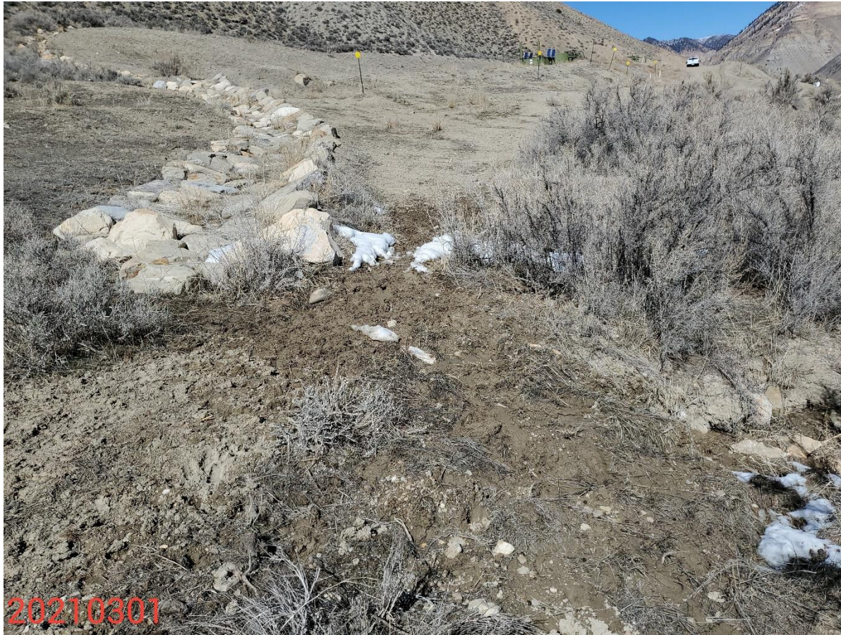
Photo 15: Photo taken from the southeastern interim areas, facing north. Photo shows areas below the sediment trap outlet where head cutting and gulley erosion degradation due to runoff is occurring.
