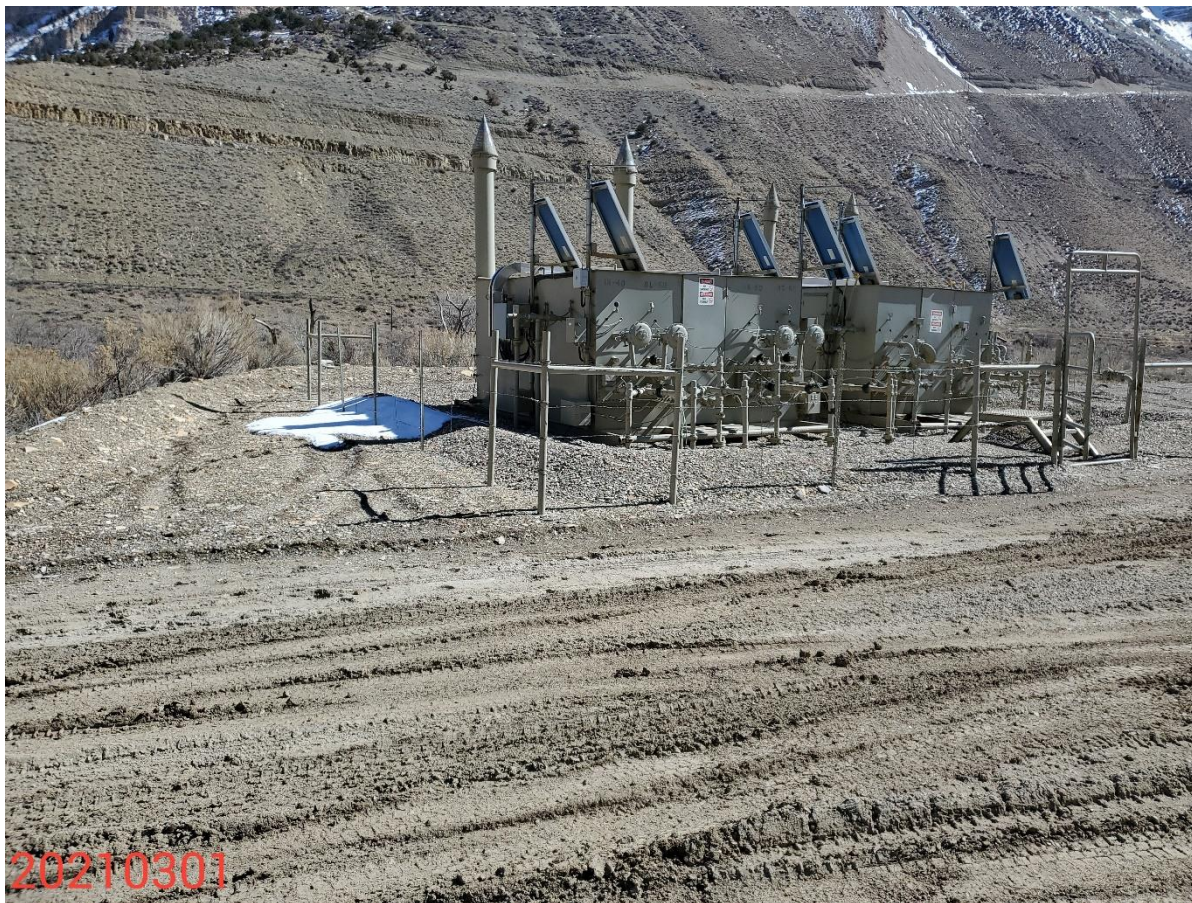
Photo 1: Photo taken from the north end of the Location, facing east. Photos 1-4 provide an overview of the Location from east, southeast, southwest to west. Photos also show control measures to stabilize production area and prevent off-location sediment transport during wet conditions has not been maintained in proper functioning condition.
