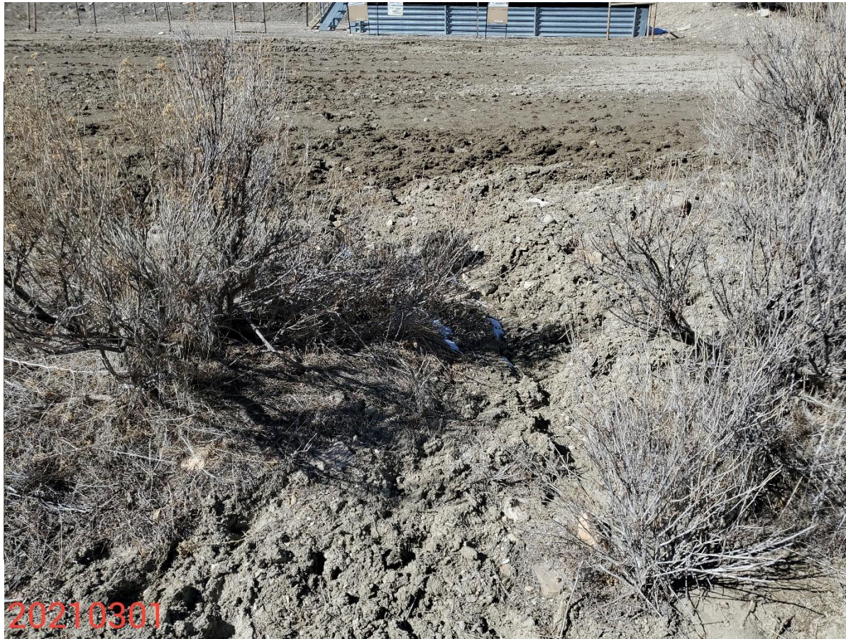
Photo 8: Photo taken from the west end of the Location, facing west. Photo shows erosion degradation due to stormwater runoff from the Location. Stormwater and erosion control measure missing or insufficient.
