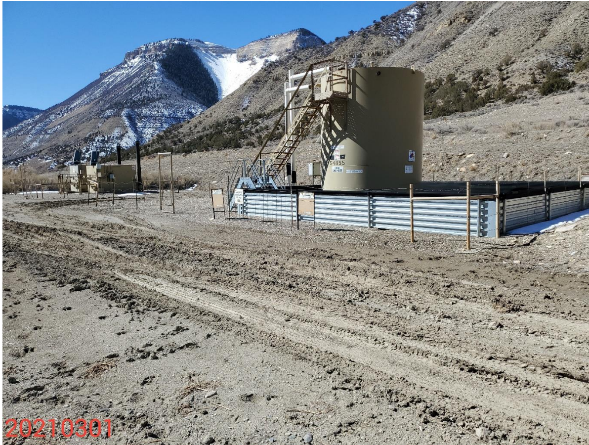
Photo 2: Photo taken from the north end of the Location, facing southwest. Photo provides an overview of the Location. Photo also shows rutting and tracking issues observed on the Location; pad not sufficiently stabilized.
