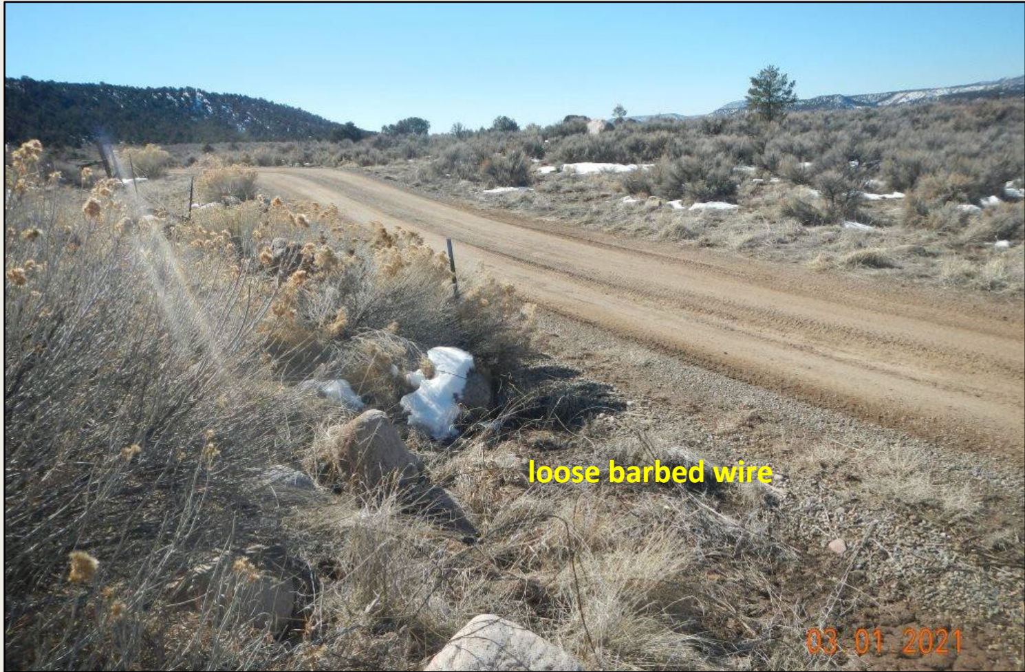
Photo 3. View of the southern project area facing eastward. Fencing is damaged and no longer functioning in many places, needing repair. Loose strands of barbed wire can be entrap wildlife.
