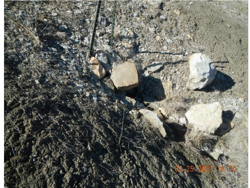
Culvert outlet basin needs maintained.
