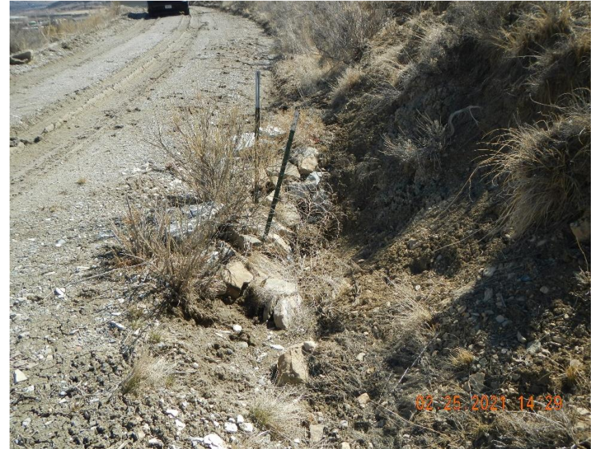
Culvert basin and ditch need maintained.
