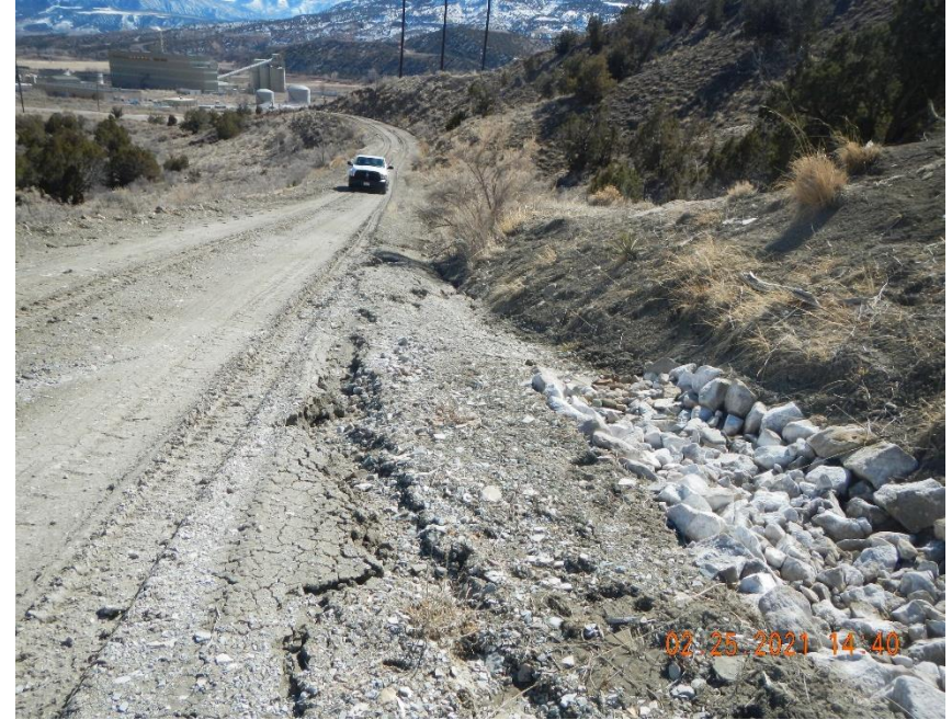
Riling from location running along ditch on access road.
