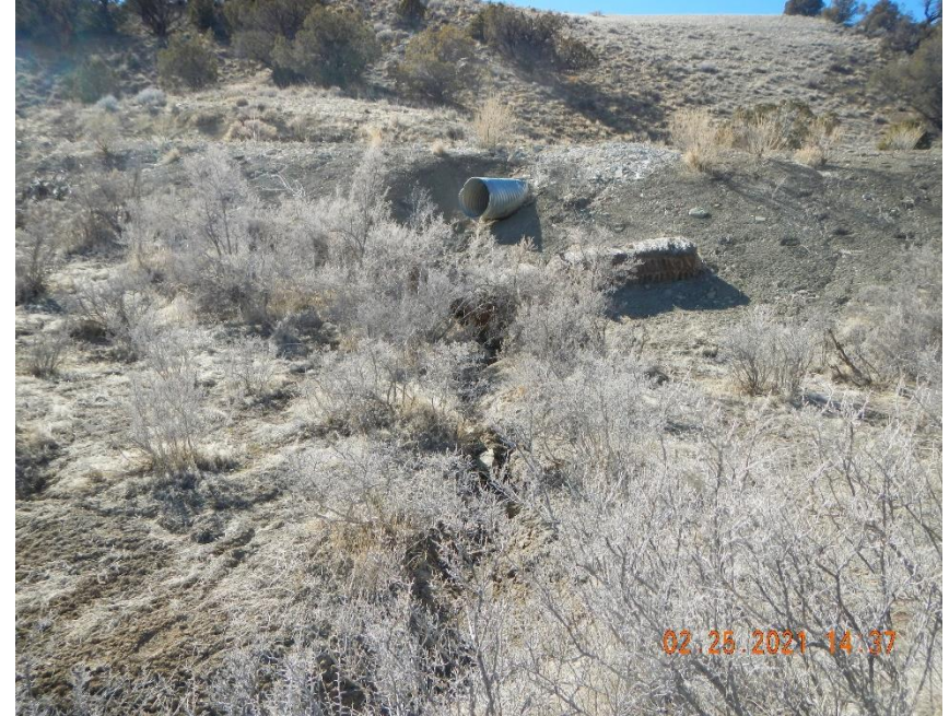
Culvert flow creating erosion rill.
