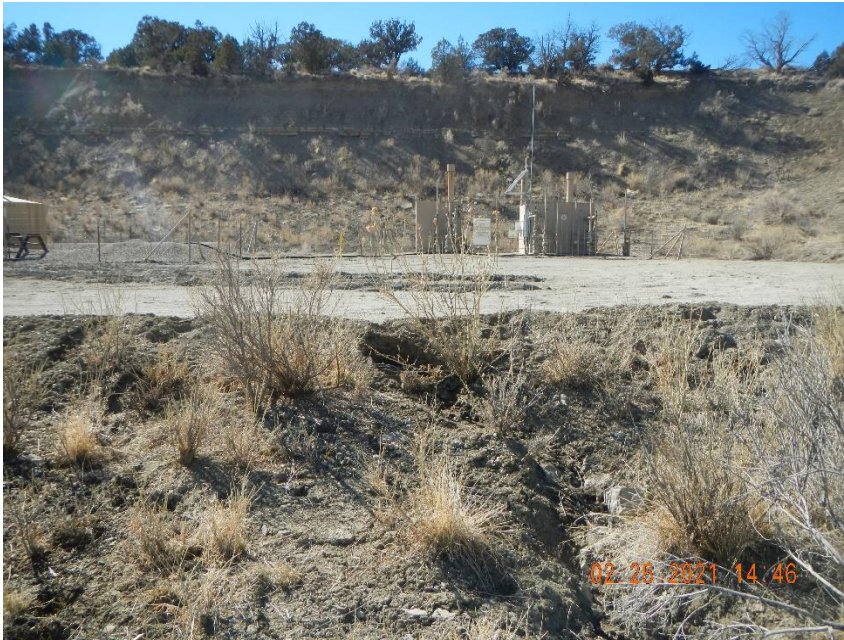
Erosion rill from channel in perimeter berm.
