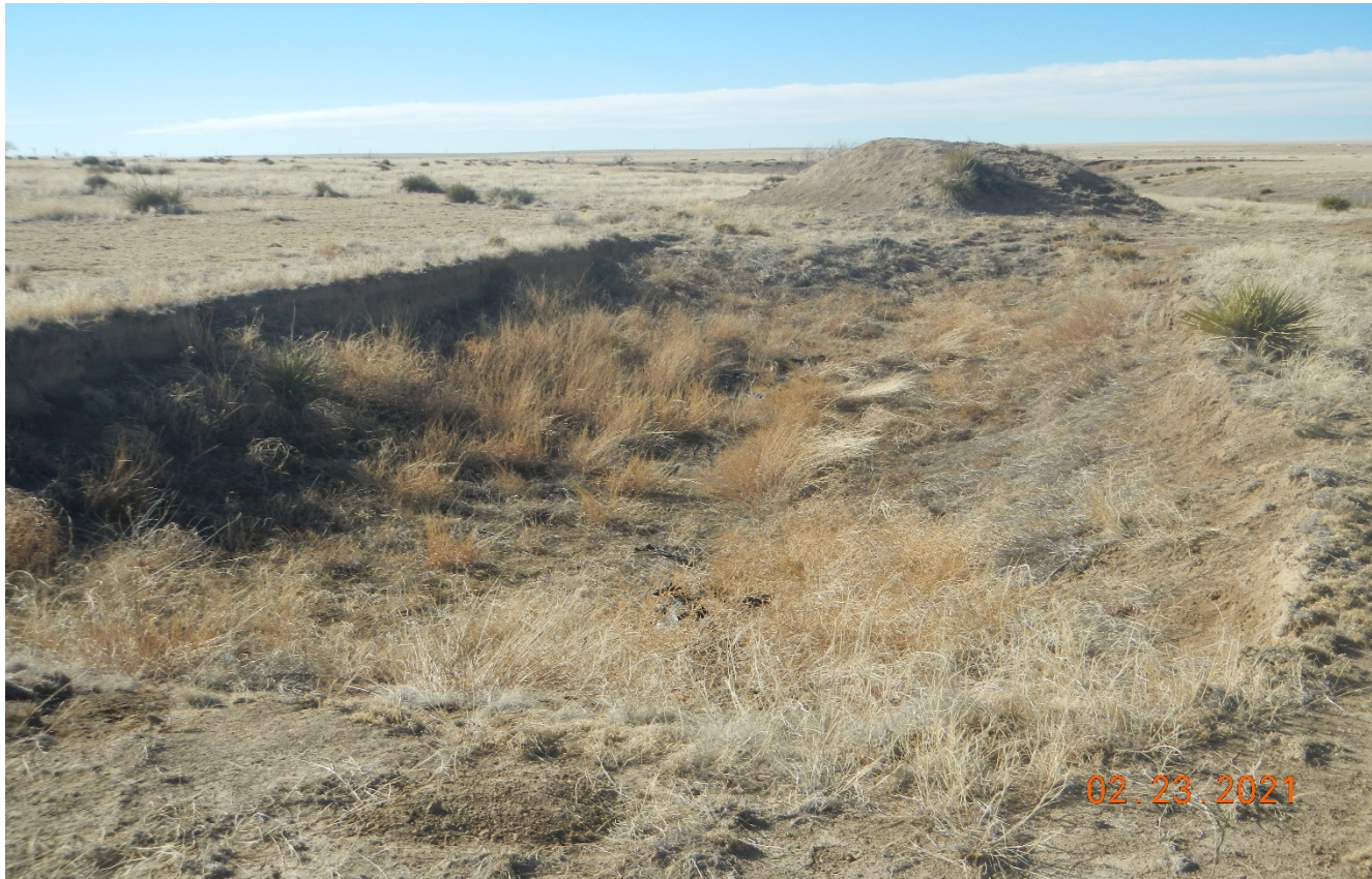
Photo 6. This pit remains at the north side of the location. Pit liner debris remains in the pit.
