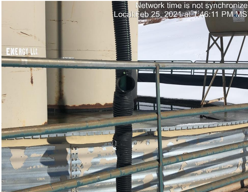
Photo #2990 Multiple flow line heating insulation open ended and not capped.
