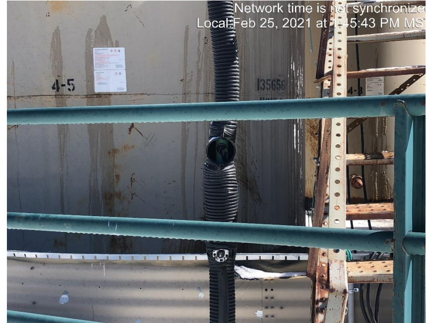
Photo #2989 Multiple flow line heating insulation open ended and not capped.
